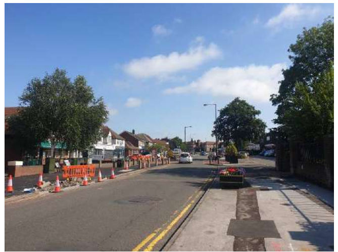
Anchor Road (view north)
