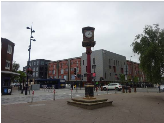
New housing on corner of High Street/Bull Street
