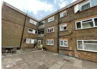
2) UPVC double glazed units have been installed to each flat. Aluminium framed units to the communal stairwell.
