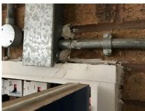
9) 1st floor service cupboard frame damaged around budget lock resulting in excessive gap & door will not secure.
