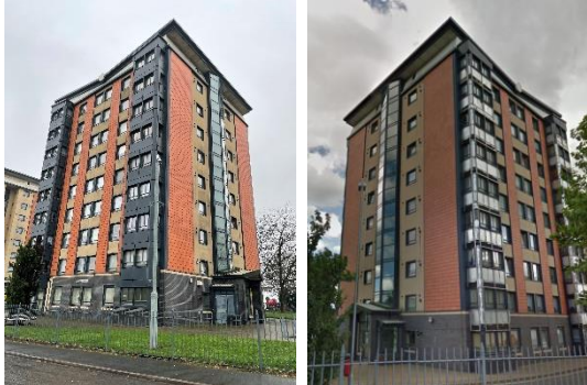
(Right – 2017 historic image showing removal of ACM)
