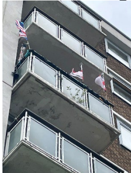
e) Flat 86 3 x flags installed to balcony.
