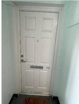
d) Flat 74 – Door fails to reliably self-close.
