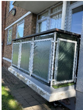
e) Flat 3 screening and netting installed to balcony.
