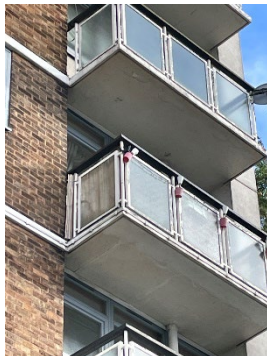
f) Flat 19 screening installed to balcony.
