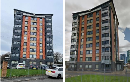
(right – 2017 historic image showing removal of ACM)
