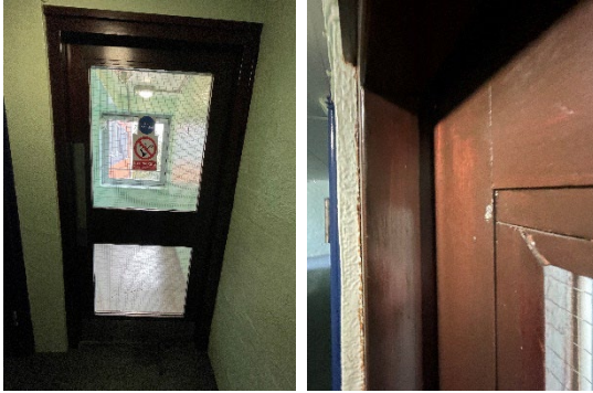
23) Floor D (3) - Communal door to stairs by flat 21 warped towards bottom of door leaf. Replacement required.
