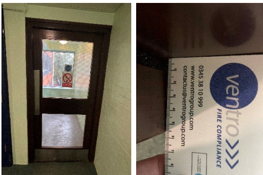
23) Floor D (3) - Communal door to stairs by flat 21 warped towards bottom of door leaf. Replacement required.
