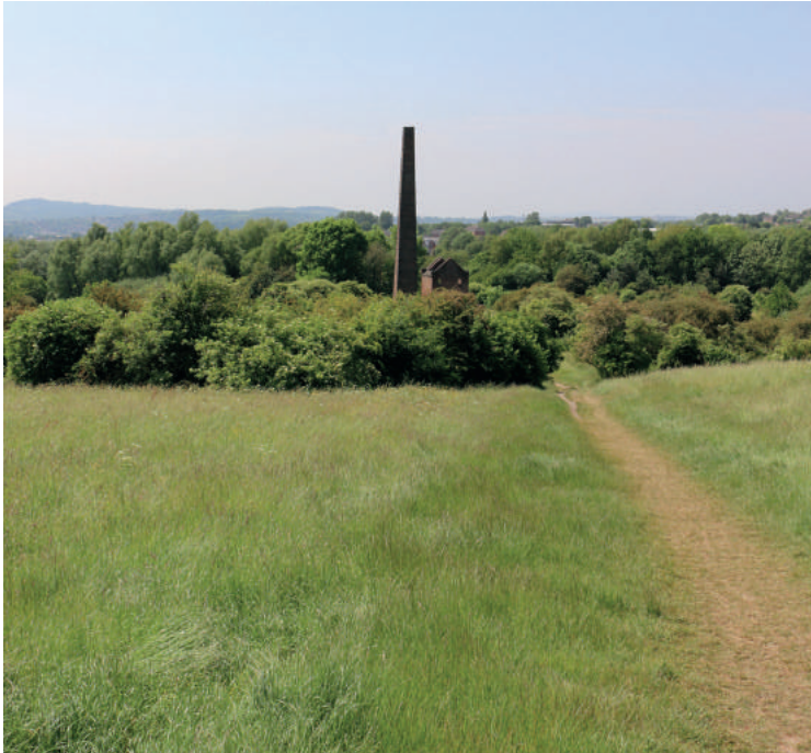
View looking south towards Cobb's Engine House and Chimney
