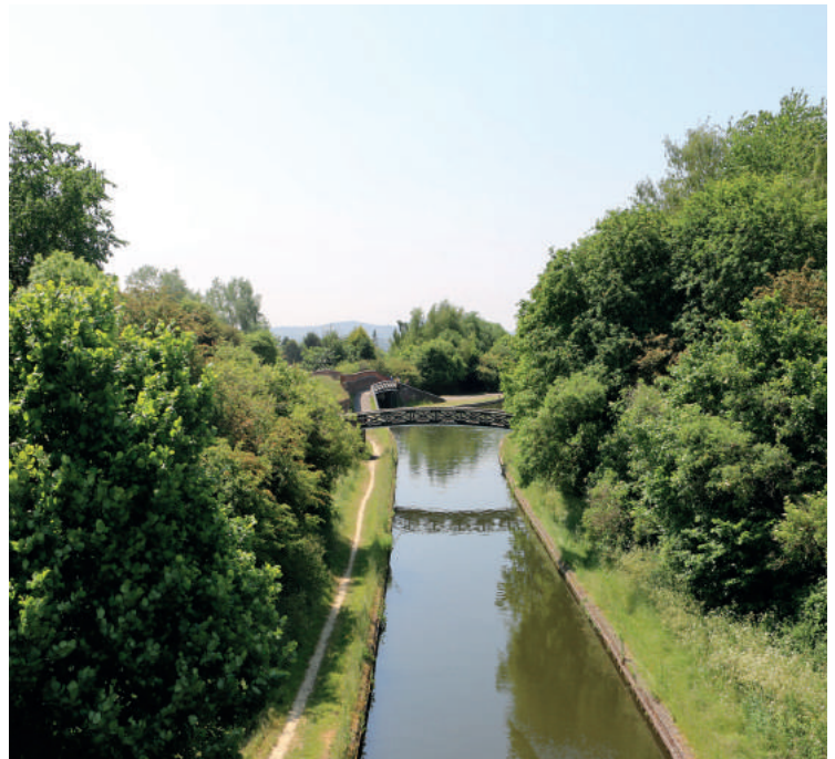
View of Netherton Tunnel Branch Canal (looking south)
