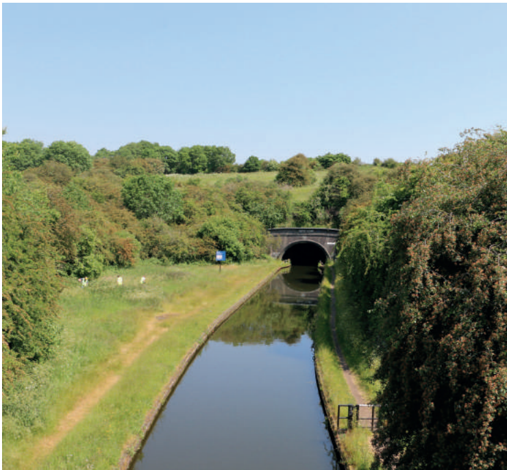
View of Netherton Tunnel Branch Canal (looking north)
