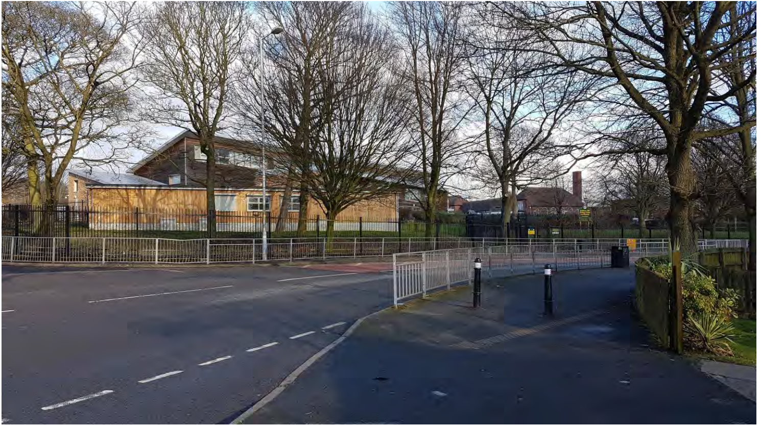
View northeast across Old Fallings Lane to school entrance.
