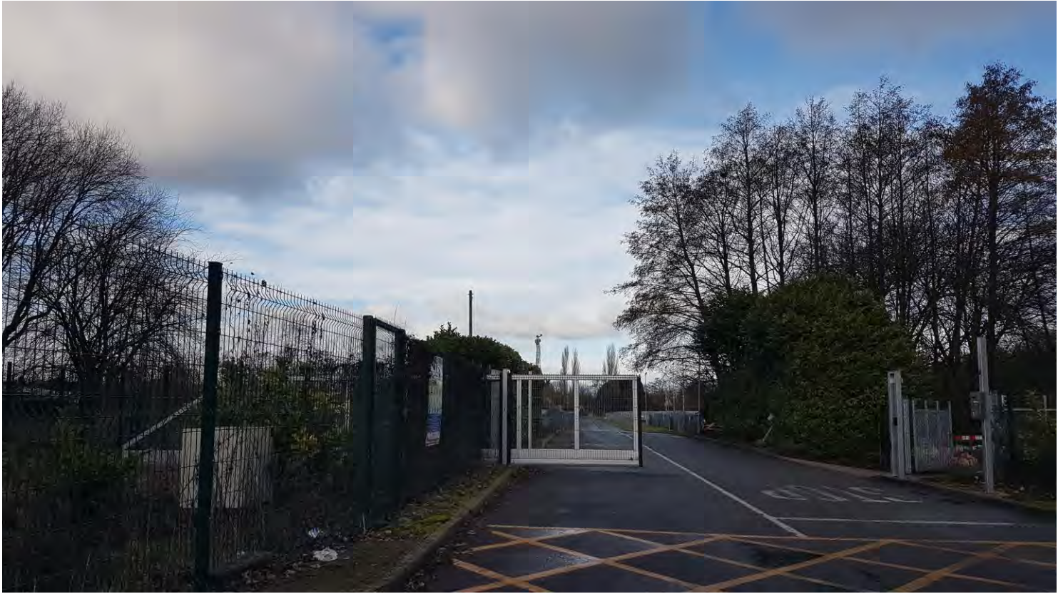
View of entrance to sewage works on Oxley Moor Road
