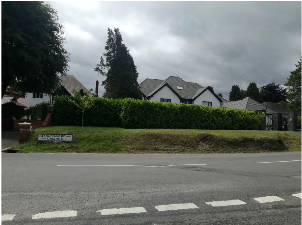
View towards dwellings on Pattingham Road; sub-parcel inaccessible and located south of dwellings.
