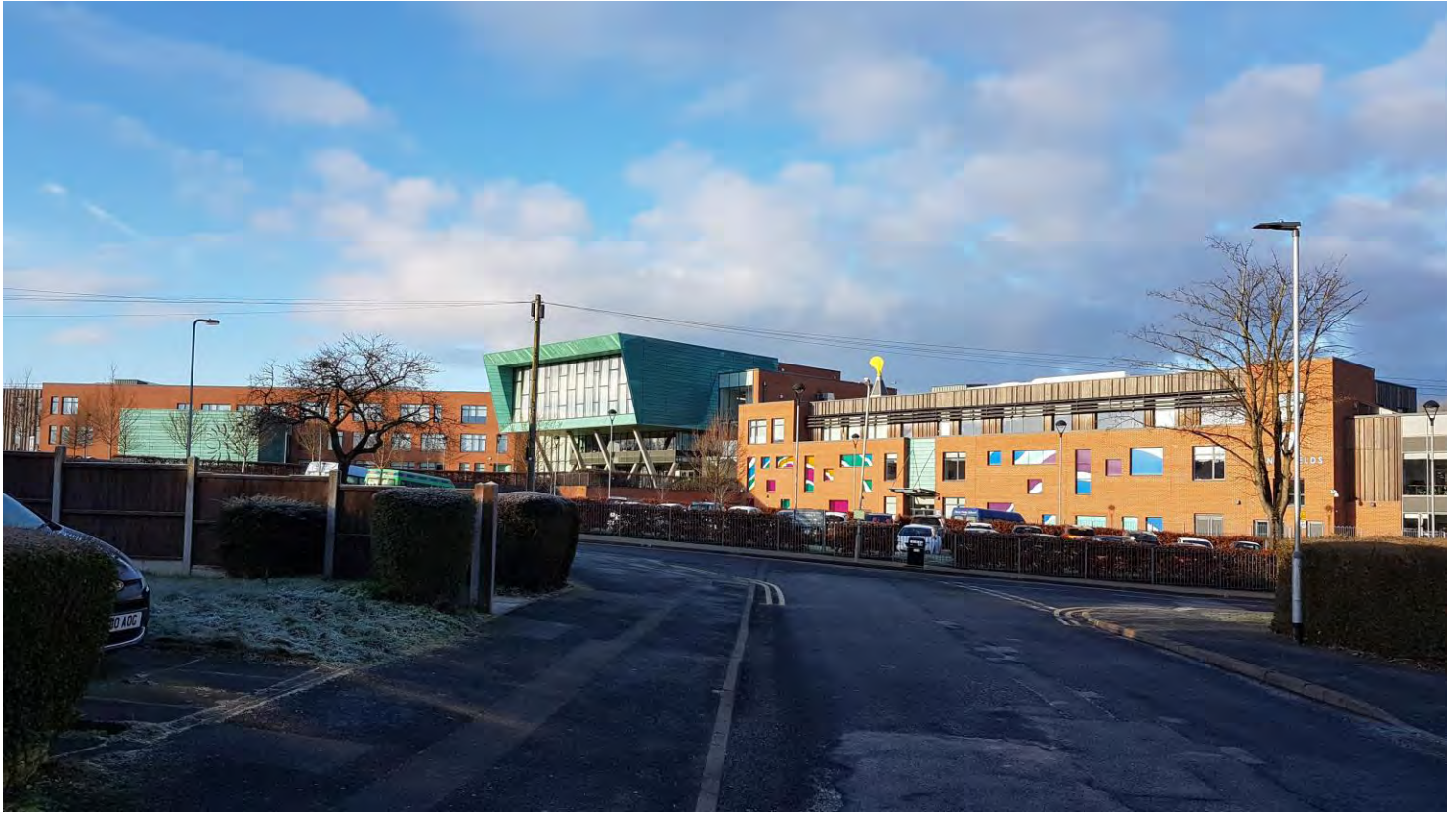
View of school buildings from entrance on Boundary Way.
