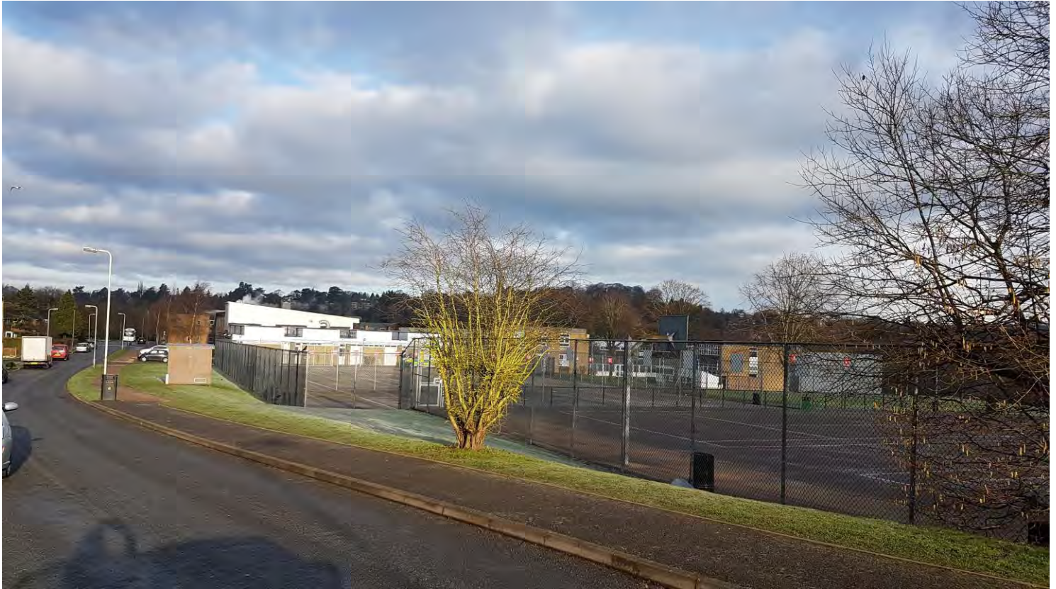
View of school buildings from Windmill Crescent.
