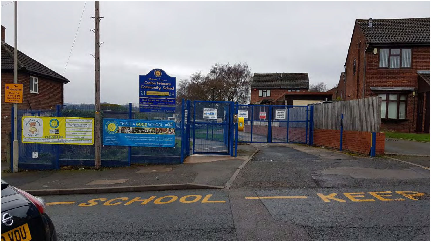
View of school entrance from Beeches View Avenue.
