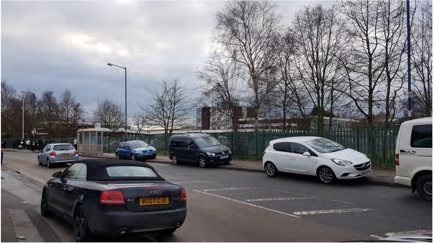
View of Bloxwich Academy from Leamore Lane.
