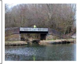
**Description:** A footbridge over the entrance to a former canal to railway interchange basin, now cut off from the canal but still filled. The bridge has blue and red brick abutments laid in English bond, rebuilt in part. The span is riveted iron with latticed parapets, painted black and white.
