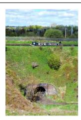
**Description:** A mid 19th century foot tunnel beneath the Birmingham New Line Canal and London & North Western railway, linking Greets Green with Tividale. The tunnel is constructed in red and blue brick laid in English
