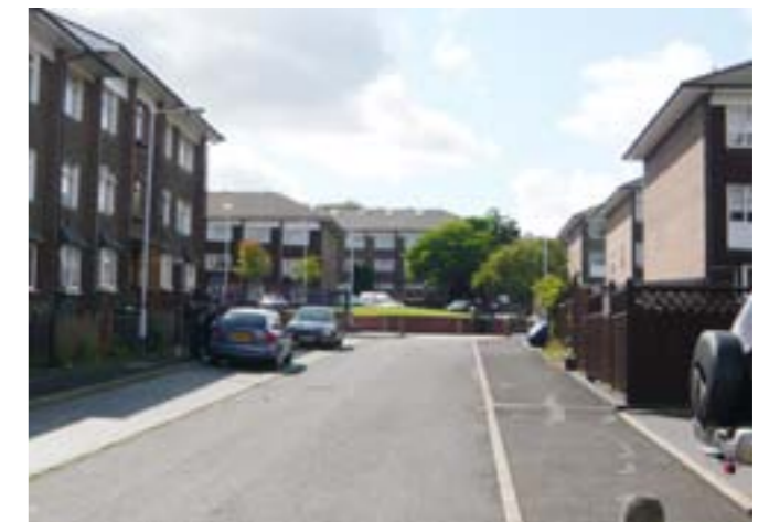
Existing view of Cuin Road Estate
