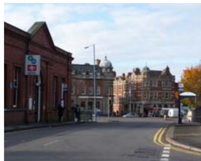
Rolfe Street Station with view to High Street
