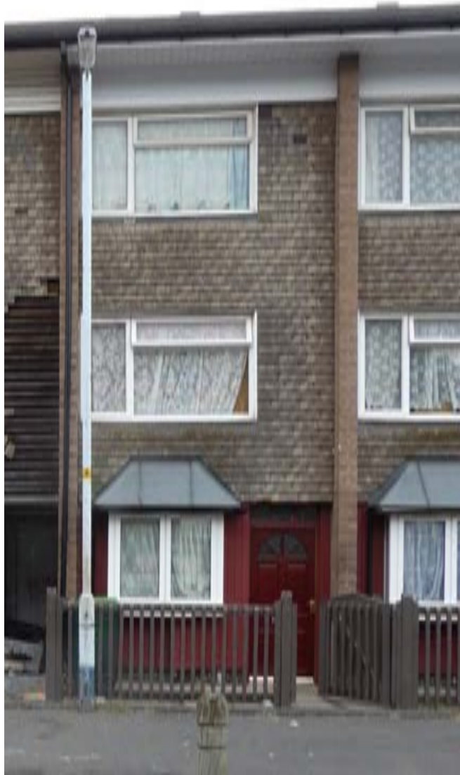
A typical narrow-frontage townhouse property
