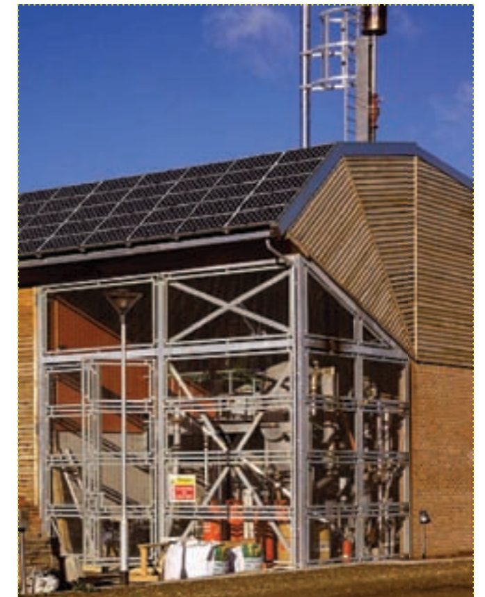
CHP plant at BedZed eco-village development
