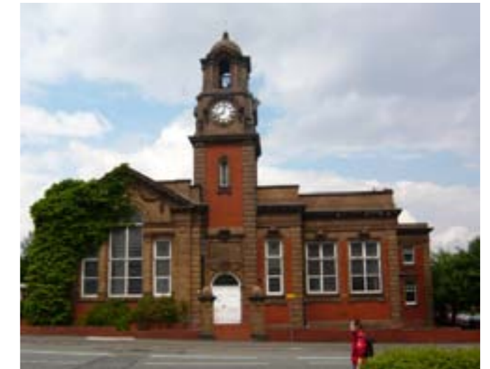
Cape House Dispensary, Cape Hill
