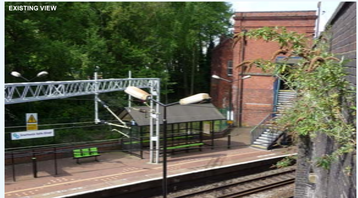
Existing view of Rolfe Street Station with secluded platforms
