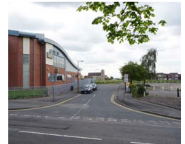
Existing view of vacant site at Windmill Precinct
