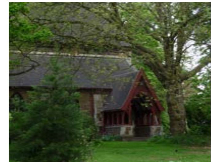
St. Matthew's Church, Windmill Lane
