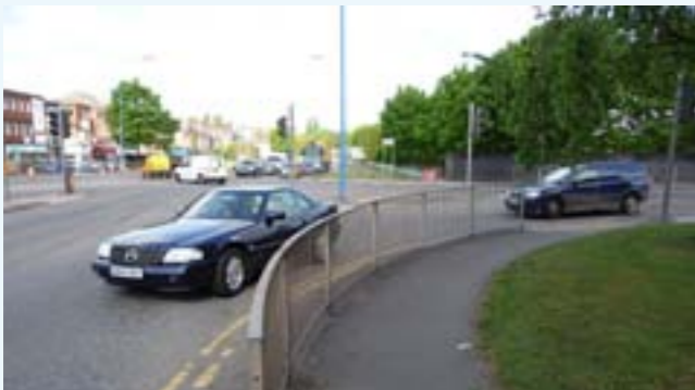
Wide-radius junction at pedestrian crossing at junction of Tollhouse Way and Rolfe Street
