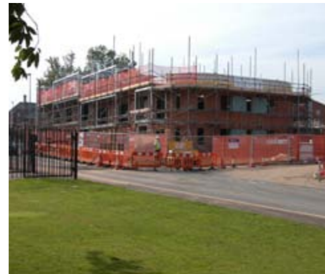
Bearwood House: New Council housing under construction
