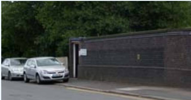
Existing view of secluded entrance to eastbound platform from Rolfe Street
