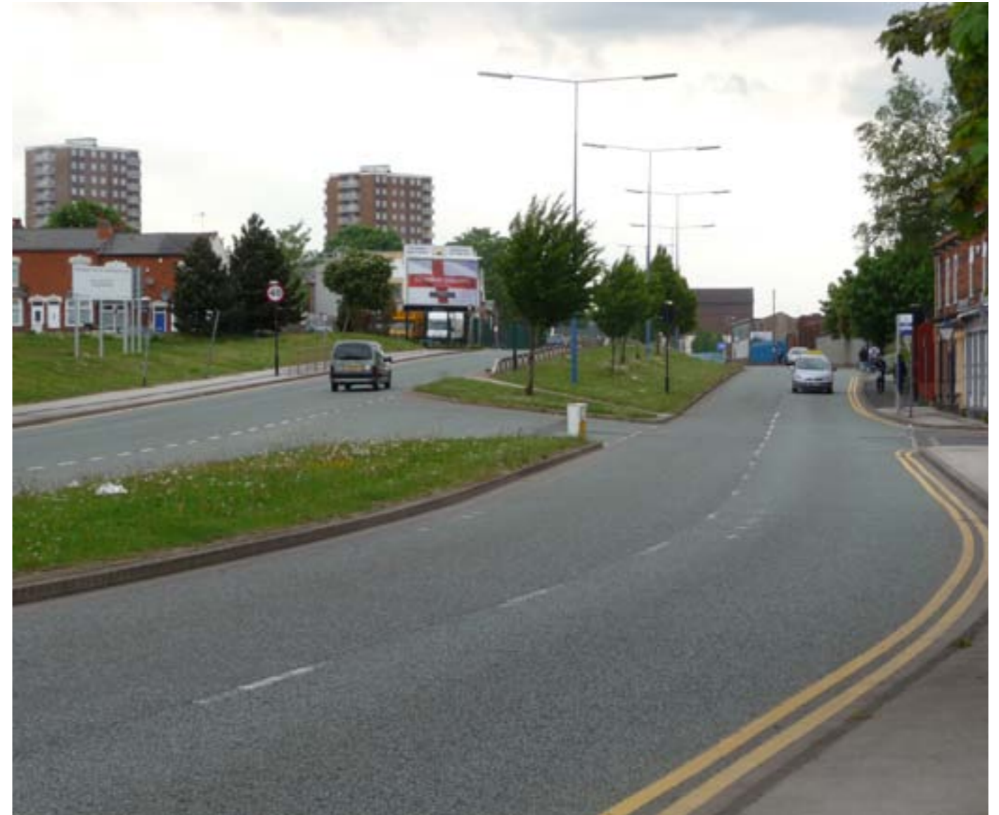
Existing crossing point at Keen Street, location of future signalised junction providing access to the new Acute Hospital site
