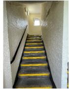
2) The means of escape are protected to prevent the spread of fire and smoke with predominately nominal Permadoor FD30s doors. No internal access to flats was gained during the fire risk assessment. Resident to flat 138 did allow an inspection of the flat entrance door. Resident confirmed smoke detection provision (not inspected).
