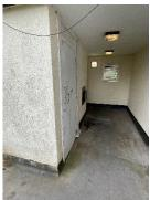
10) Flat 126, ground floor, has a rear door that opens into the staircase. This is a UPVC door and should be replaced with a certified self-closing FD 30s door set. This has been noted in the observation section and an email sent to the project manager of the door programme. The door presents a low risk as the staircase is not enclosed and this is the only door onto the staircase.
