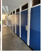
10) The panel above the store doors, within the staircase, offers no fire resistance as a steel mesh construction. The panels should therefore be infilled with a fire resisting panel.
