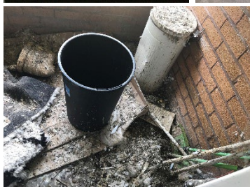
(Balcony without netting Block 17-23)
