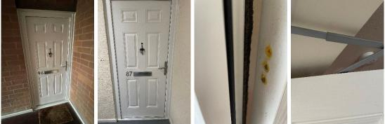
3) The only communal doors within the block are the final exit doors and doors into the drying area which are fitted with automatic closing devices that are checked on a regular basis by the Janitorial Teams as part of their daily checks.
