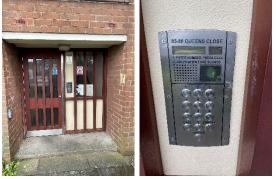
Each main entrance has a door entry system with a firefighter override switch.
