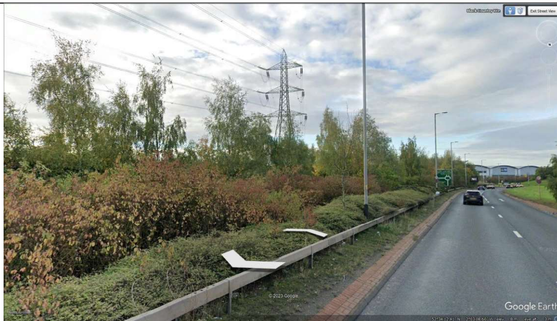
Location - Black Country Route, approaching Lunt Junction westbound Lamppost 22
