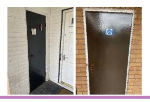
10) Flat entrance door 52 is scheduled to be changed to a certified self-closing FD 30S as confirmed by door programme manager. This door is located at the end of the block and is not on a travel route therefore is of low risk.
