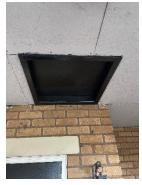
9) Store doors located next to flat entrance doors and to underside of staircase should be considered for upgrading works to certified FD 30s door sets during the next future works programme.
