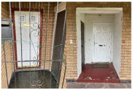
3) Brickwork, on external escape route, is approx. 1300mm to bottom of window. This is deemed acceptable for a person to crouch and pass the window. Please note a stay put unless strategy applies to this building.
