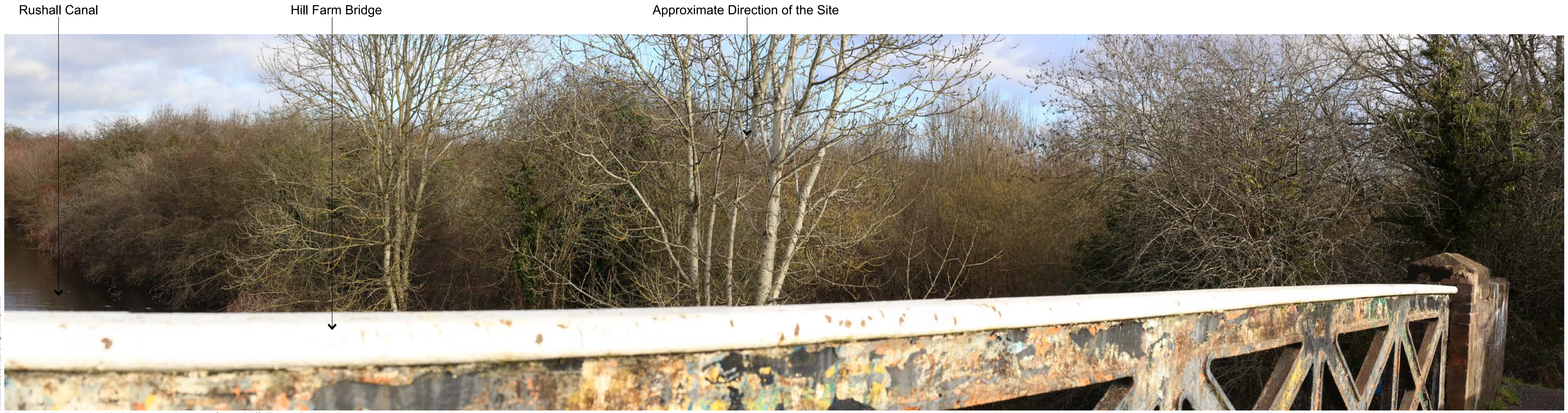
Photo Viewpoint 6: View north-east from Hill Farm Bridge
