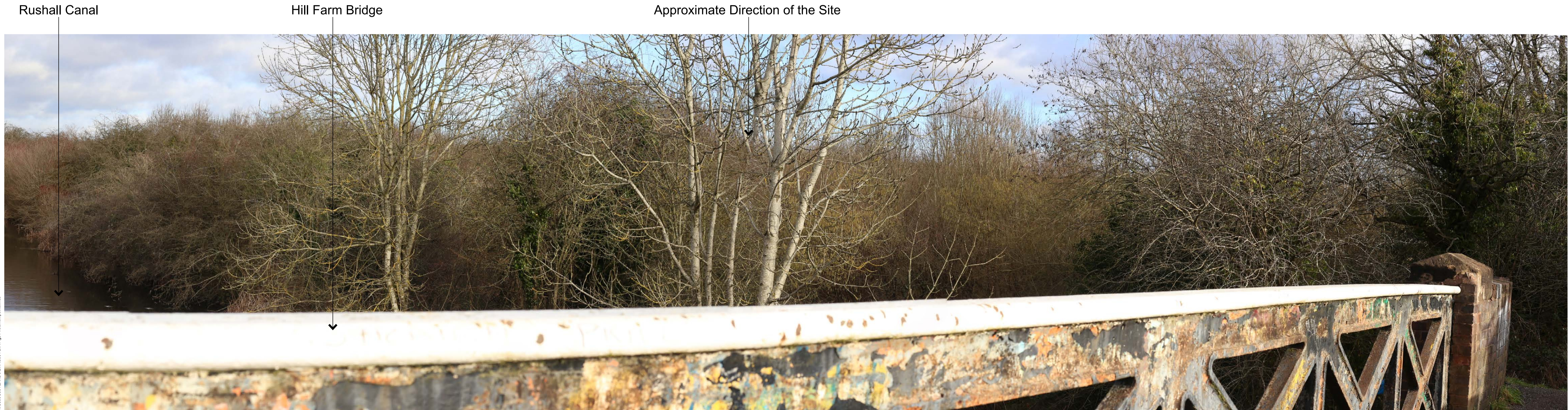
Photo Viewpoint 6: View north-east from Hill Farm Bridge
