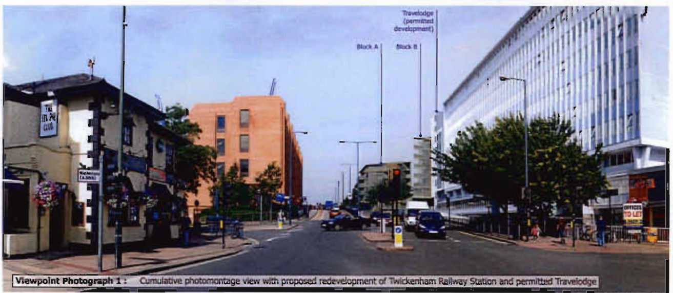
Figure 8.3 Cumulative photomontage of redevelopment at Twickenham Railway Station with other permitted development, a neighbouring hotel extension. Note the aspect ratio of the image to encompass the vertical field of view of the urban context; camera used in portrait orientation
