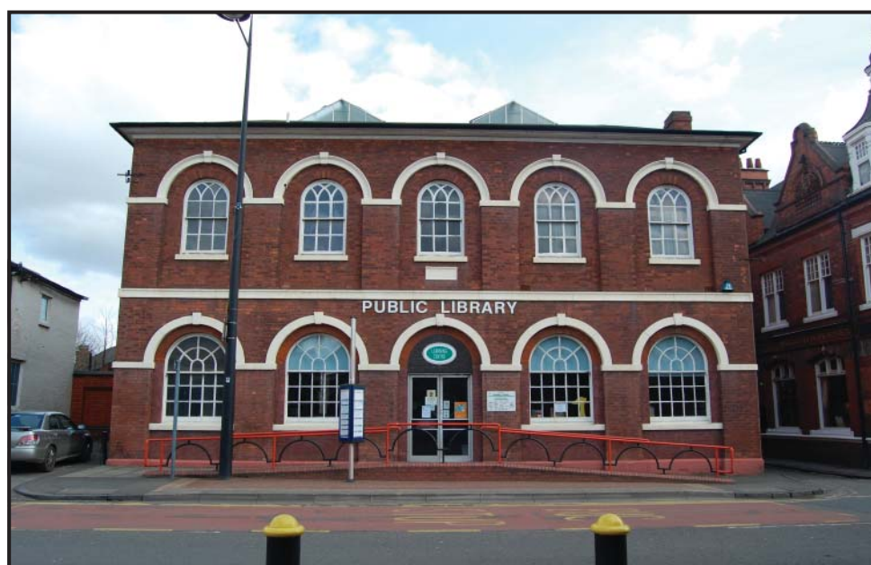
Plate 20: Oldbury Public Library, Church Street.
