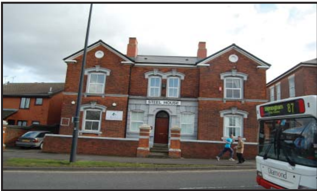
Plate 35: Steel House, Church Street.
