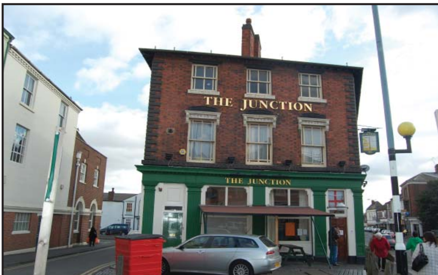
Plate 42: The Junction Public House, Birmingham Street.
