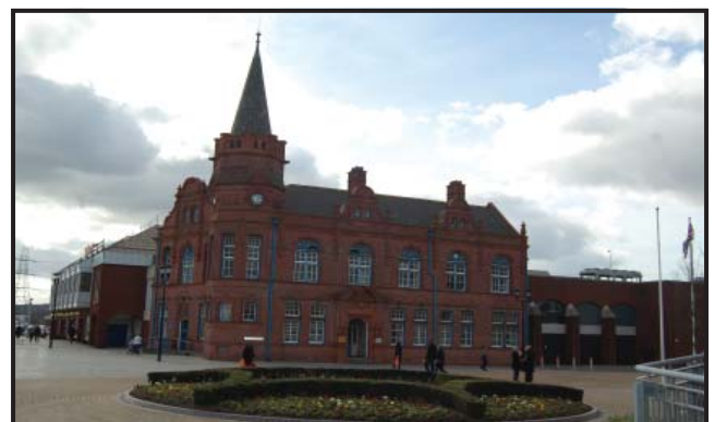
Plate 38: Former Public Library, Freeth Street.
