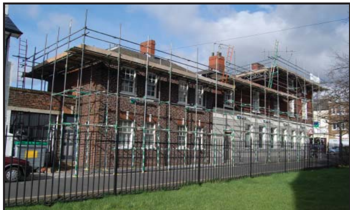
Plate 55: Renovations of Lloyds Bank, Church Square.
