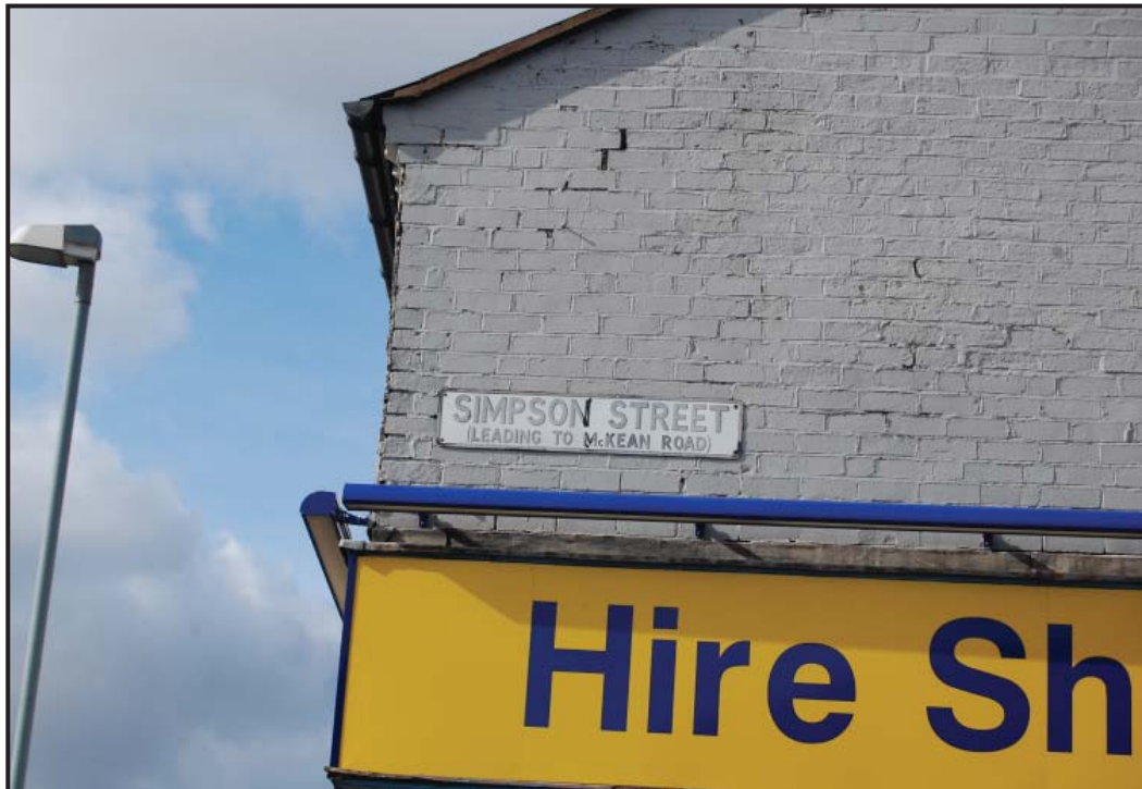
Plate 59: Inappropriate Signage, corner of Simpson Street.
