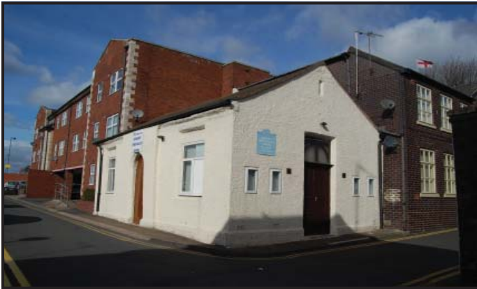
Plate 27: Former Baptist Chapel/Schoolhouse, Canal Street.
