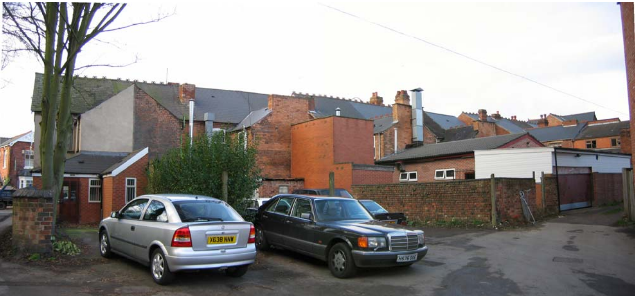
Plate 20: View from Victoria Avenue of the backs of the terrace on the east side of High Street
