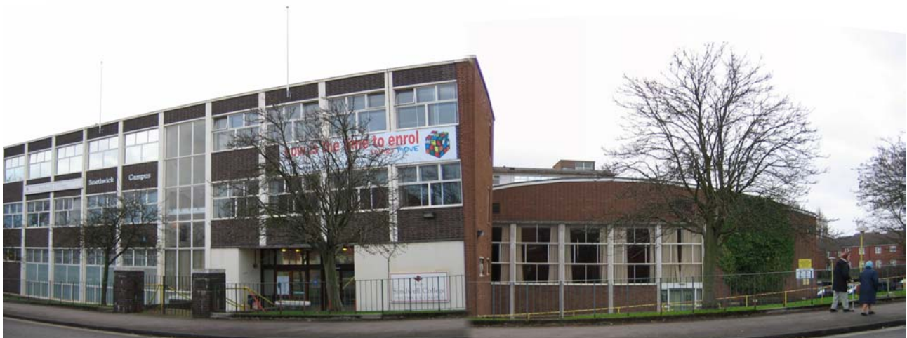
Plate 50: Modern Smethwick College buildings
