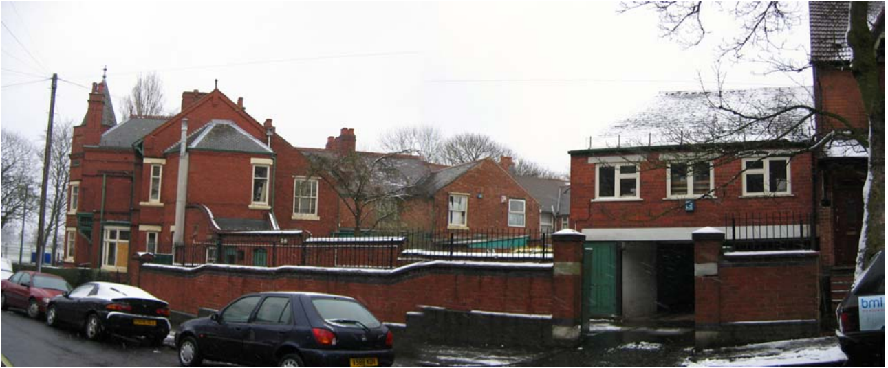
Plate 47: No. 368 High Street, boundary wall and former coach house, Edgbaston Road
