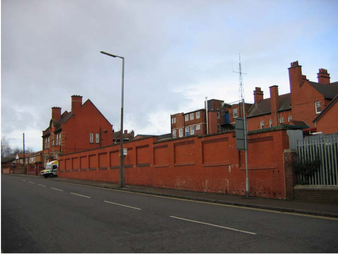
Plate 5: Boundary wall to rear of police station on Crocketts Lane
