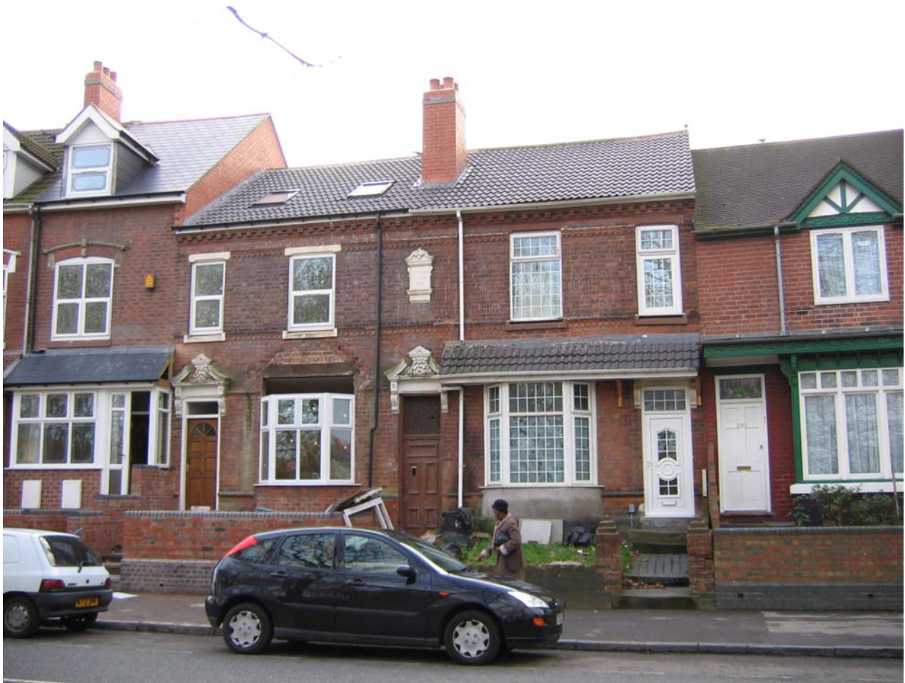
Plate 49: The paired villas of the 1880s, at the east end of the terrace Nos.370-80 High Street, showing the extent of alterations to the front elevations
