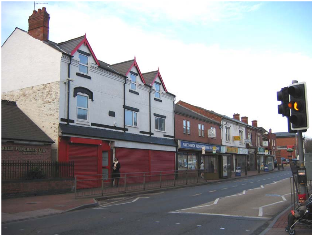
Plate 12: Nos. 262-278 High Street (west side)
