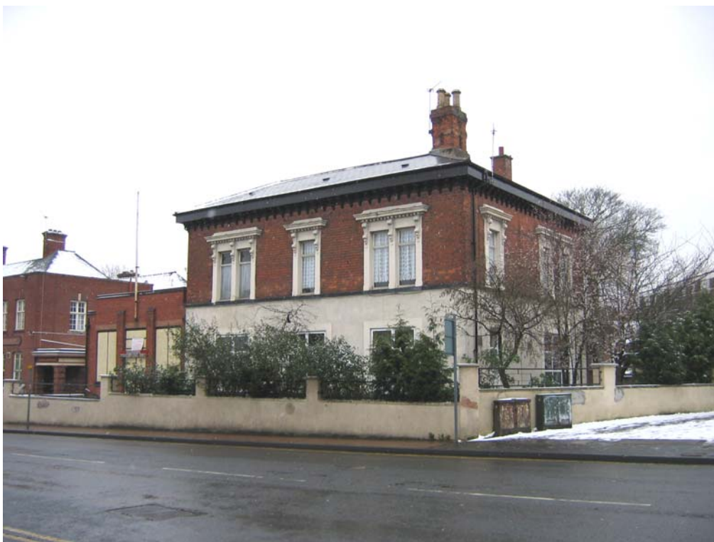
Plate 10: Nos.236-240 High Street, west side (Smethwick Conservative Club)
