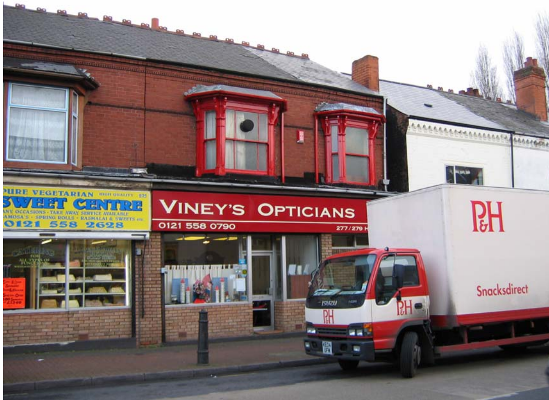
Plate 15: Canted bays above Viney's Opticians, Nos. 277-279 High Street (east side)
