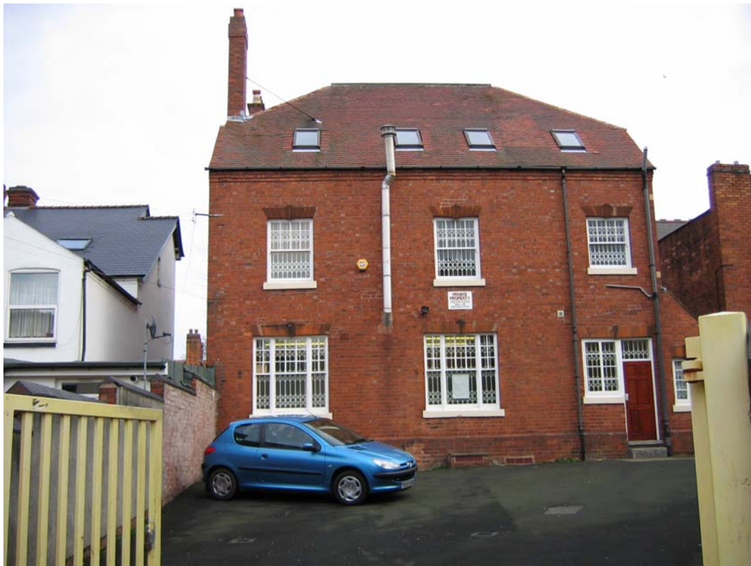
Plate 36: Rear elevation of No. 2 Bearwood Road
