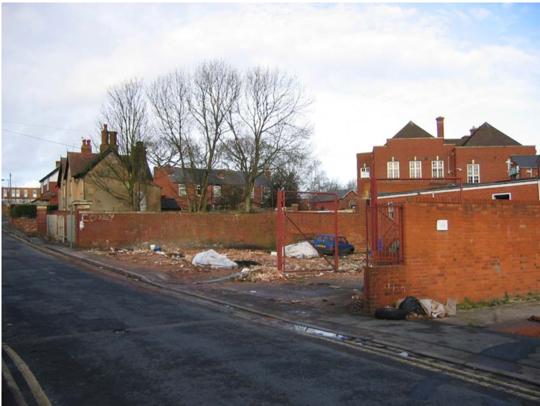
Plate 52: Site of the now-demolished Nos. 128-130 Firs Lane
