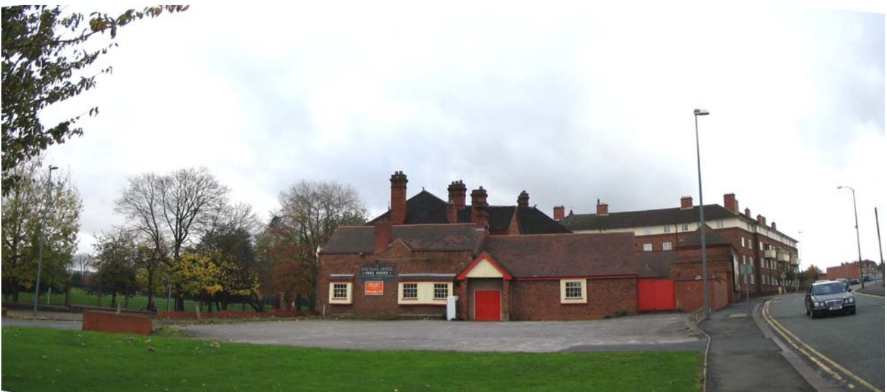
Plate 40: Car park and north elevation of The Park Hotel
