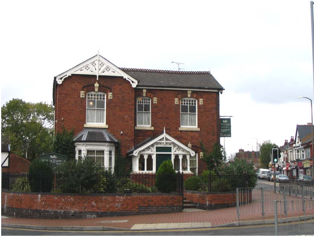
Plate 21: Maben House, No. 280 High Street (corner of Firs Lane)
