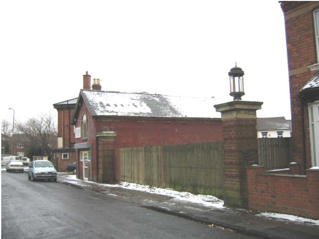
Plate 26: The Red Cow gate piers on Arden Road
