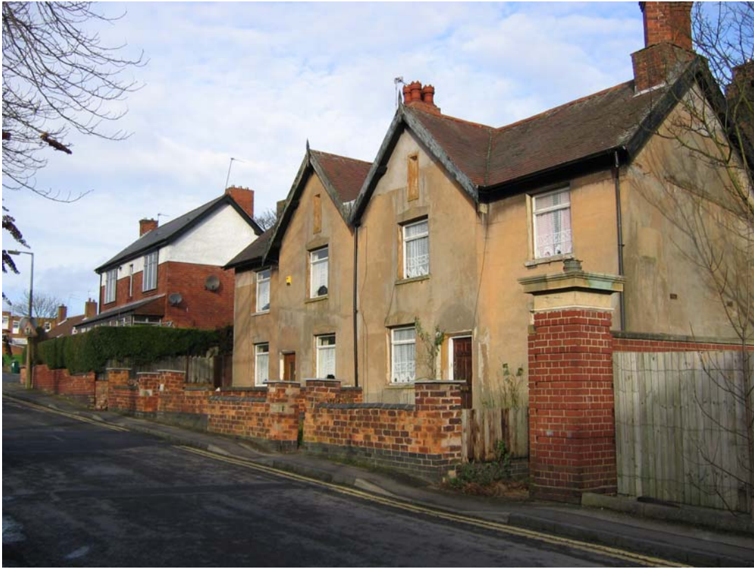
Plate 23: Late Victorian Cottages, Firs Lane (east side), with Red Cow gate pier in right foreground
