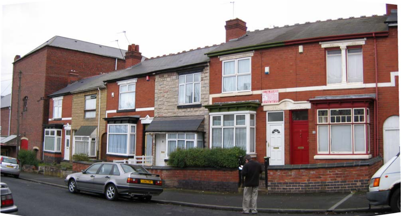
Plate 1: St. Alban's Road, southeastern side
