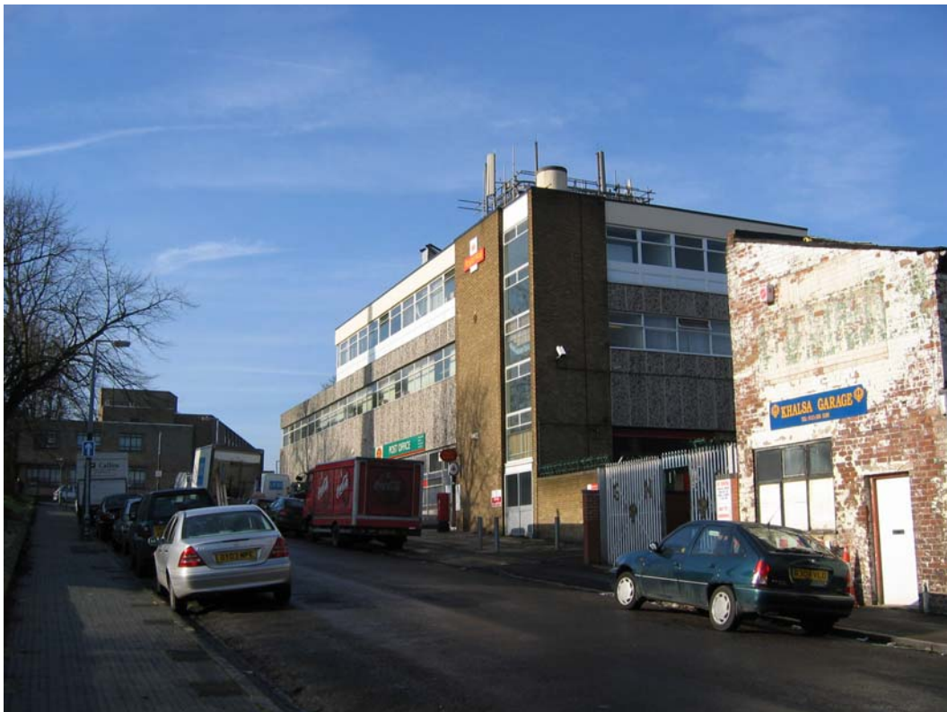
Plate 34: Post Office building on Trinity Street
