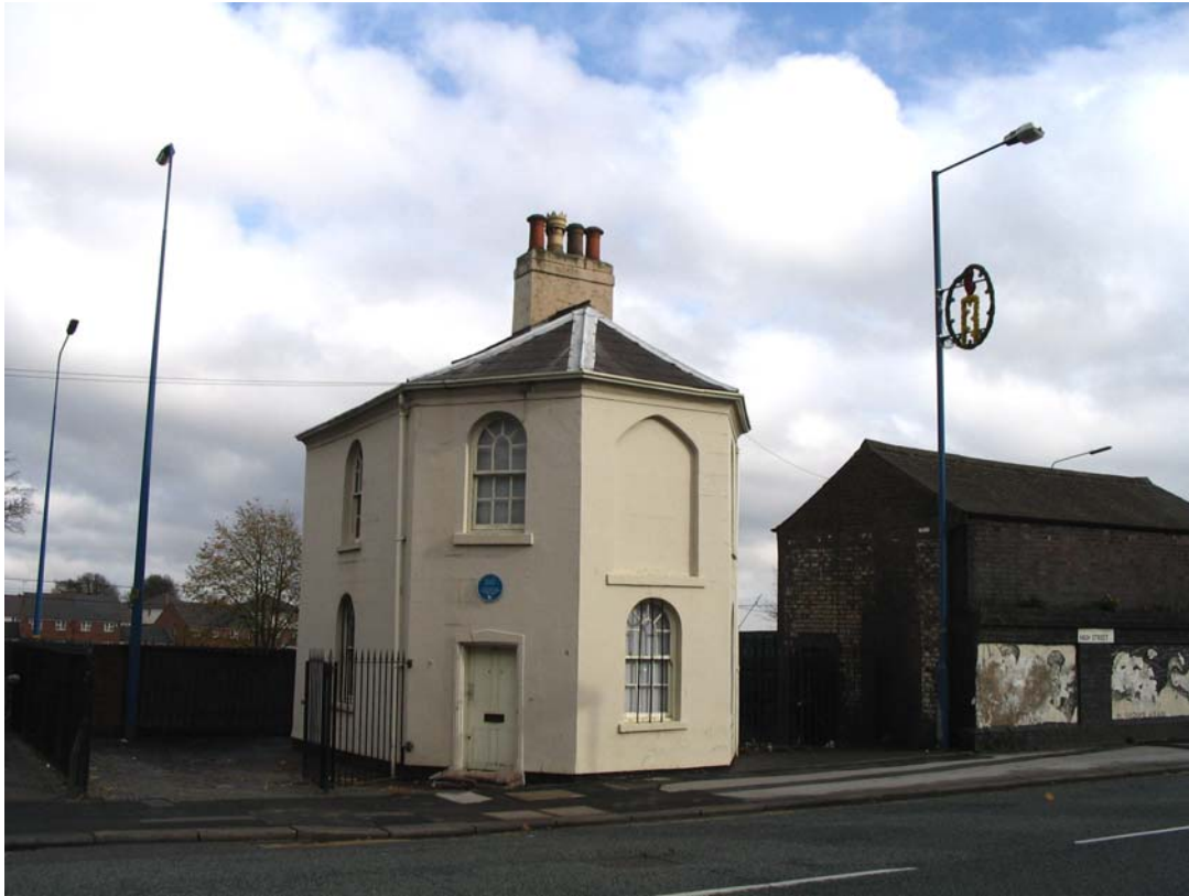
Plate 27: The Toll House and former railway shed
