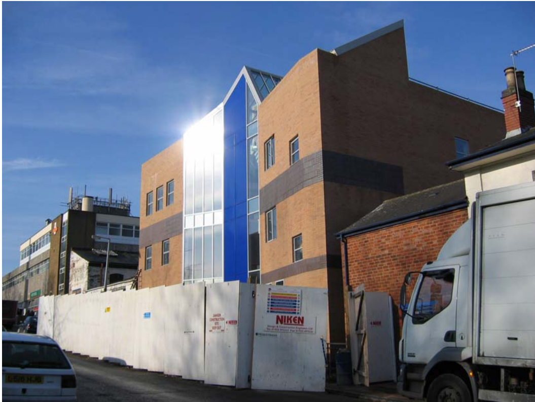
Plate 35: New building under construction on Trinity Street
