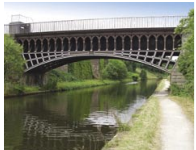
Engine Arm Aqueduct
