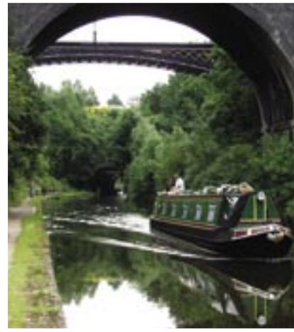
New Main Line - Rail Bridge with Galton Bridge behind
