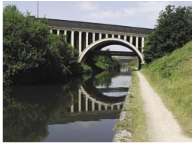
Spon Lane South Bridge, 1829. Widened 1927.
