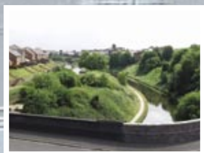
View from Brass House Lane Bridge 2003
