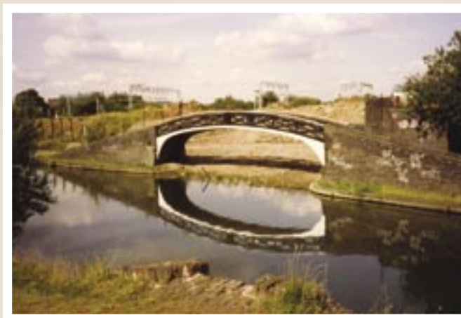
Former Soapworks Basin Bridge
