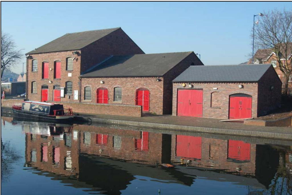
Plate 8: Old Malthouse Stables.
