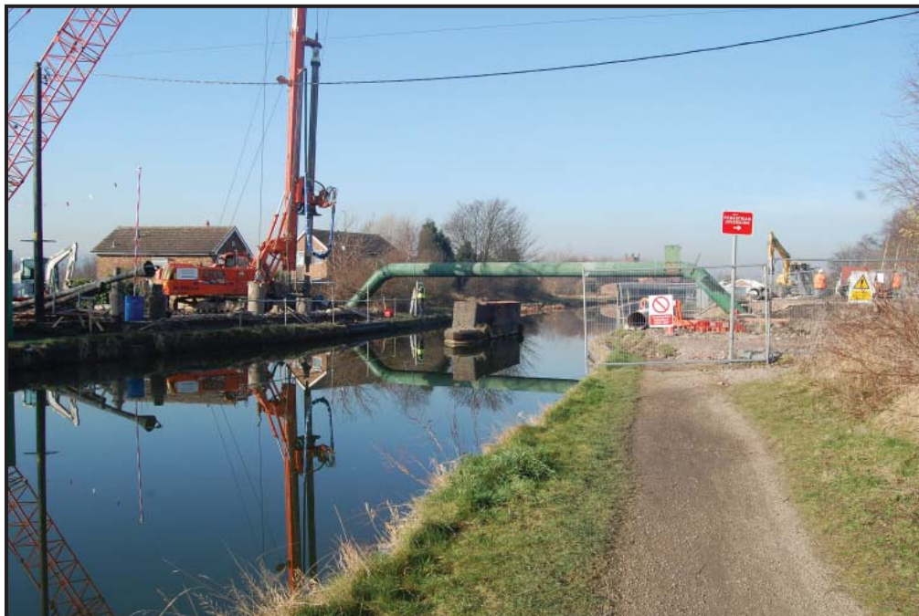
Plate 51: Watery Lane Bridge.
