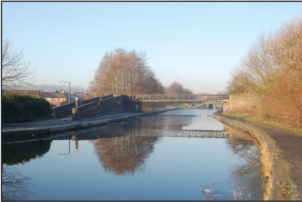
Plate 3: Wood Street Footbridge.
