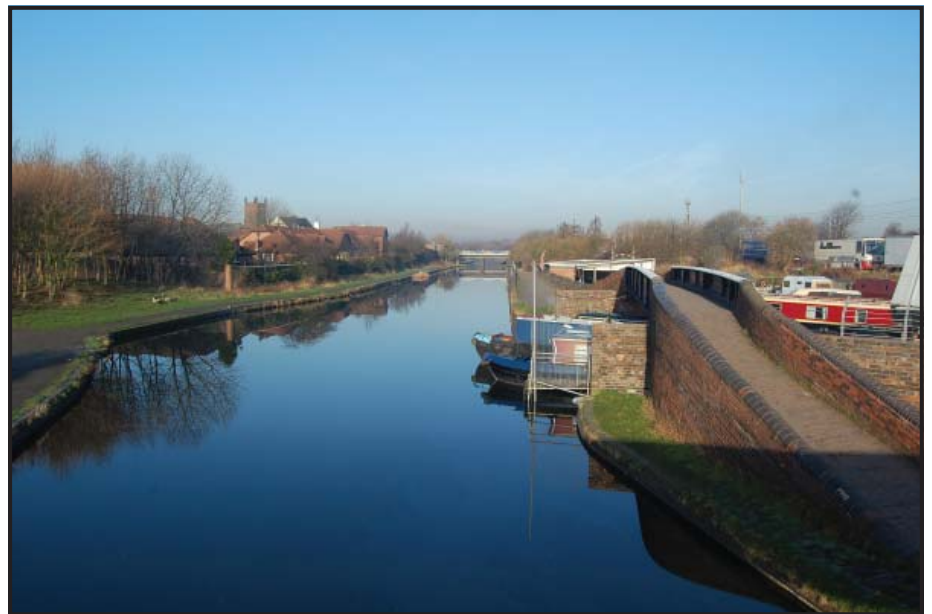
Plate 11: New Line from Waterloo Road Footbridge.
