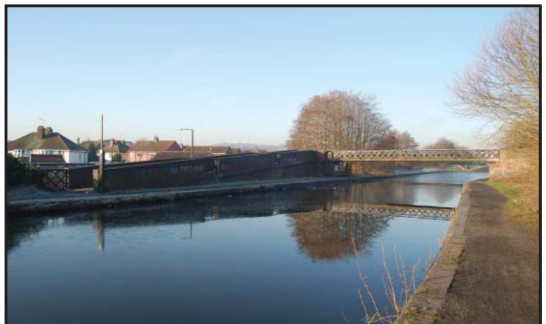
Plate 27: (1) Wood Street Footbridge.
