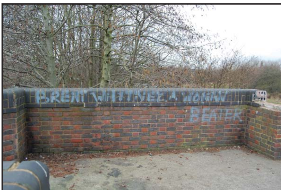
Plate 48: Wood Street Footbridge.
