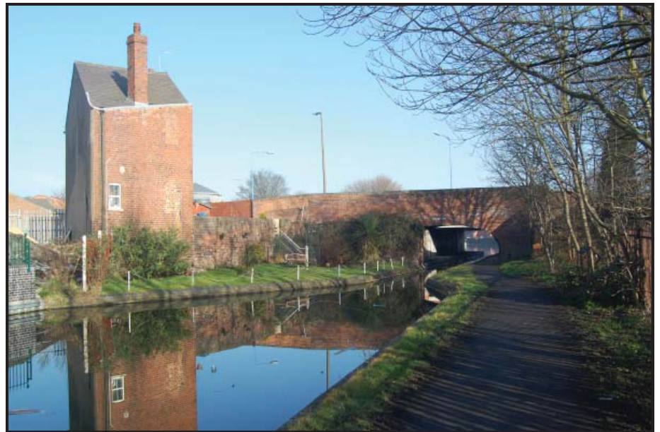
Plate 14: Tipton Green Bridge from the South.
