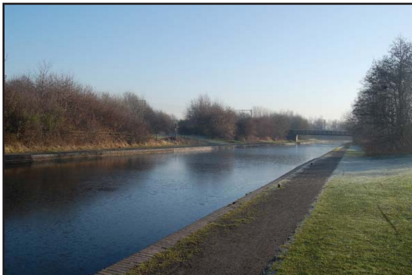
Plate 18: New Line from Waterloo Road Footbridge.
