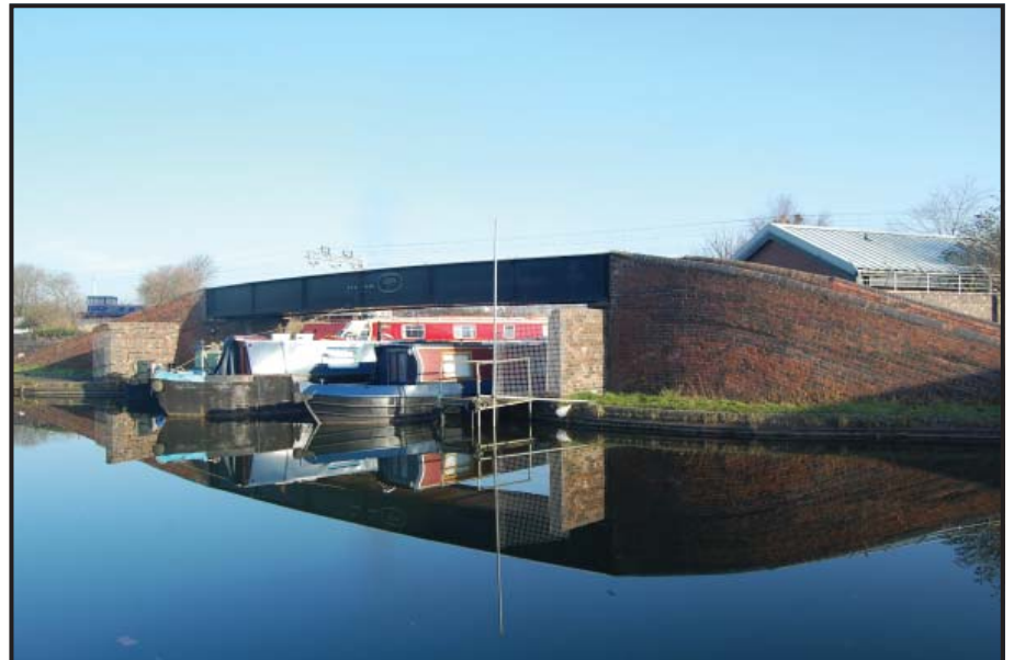
Plate 32: (15) Toll End Communication Canal Roving Bridge.
