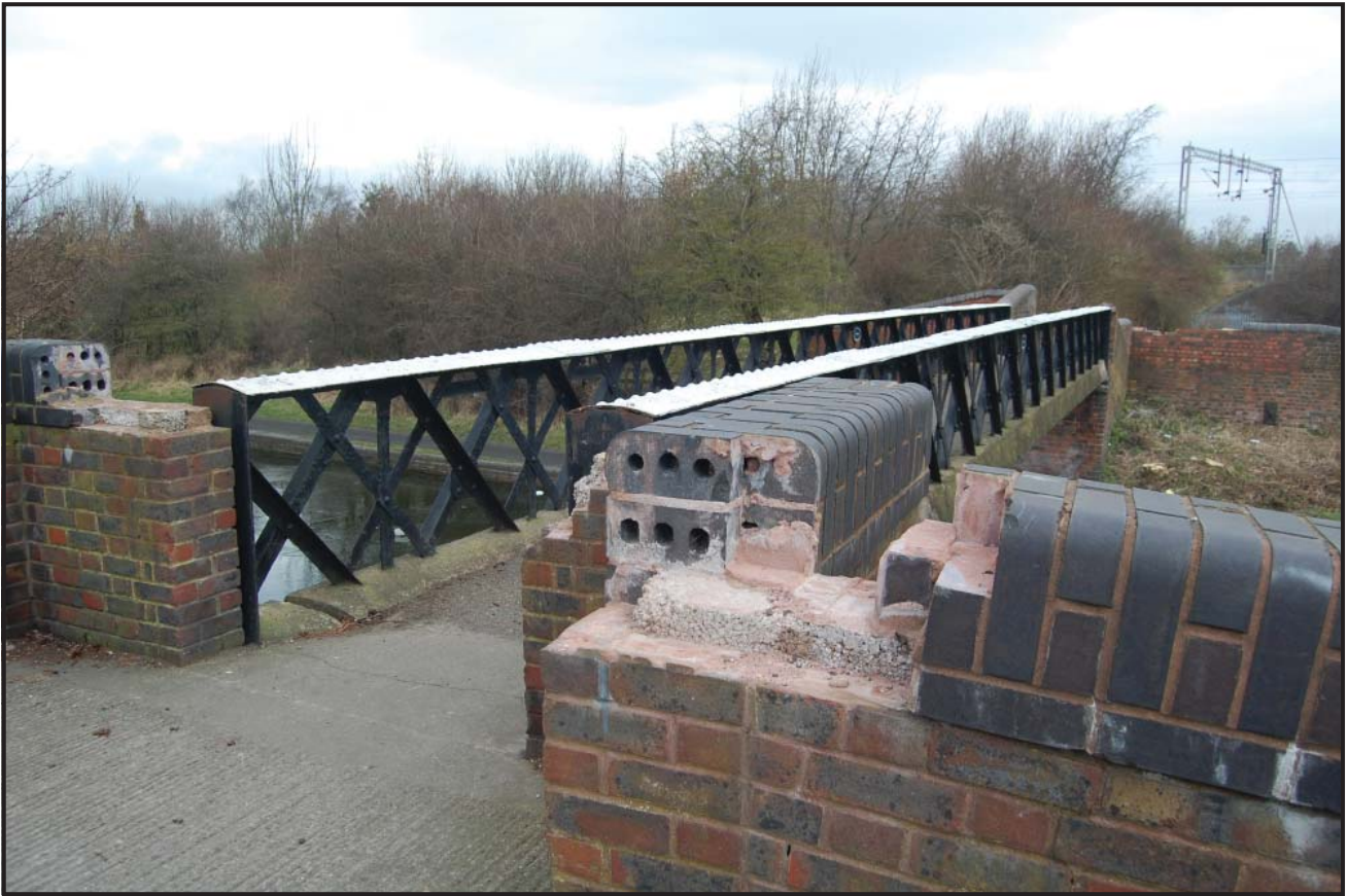
Plate 57: Wood Street Footbridge.
