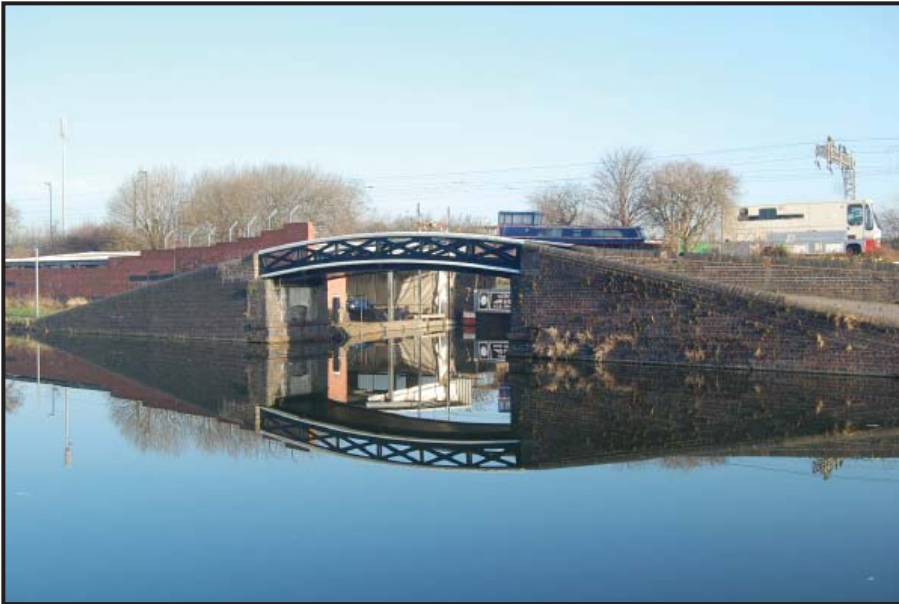
Plate 31: (14) Cast Iron Footbridge Approx. 150m West of Waterloo Road.
