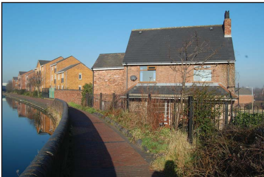
Plate 39: (19) Canalside House, Factory Road.
