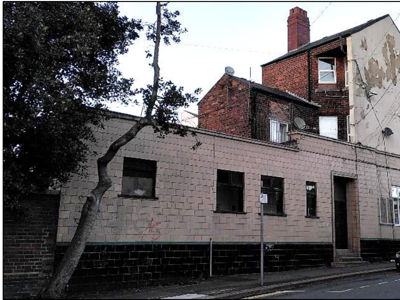
Figure 78 Rear extension of 8 Market Place, facing onto The Shambles.
