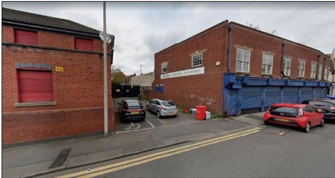
Figure 70 Gap site Russell Street. Google Streetview.
