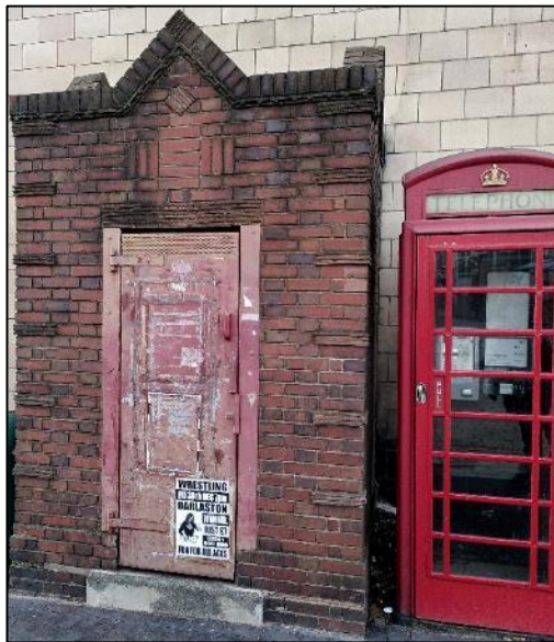
Figure 60 Former telephone or exchange box, locally thought to have been a Police Box, Shambles.
