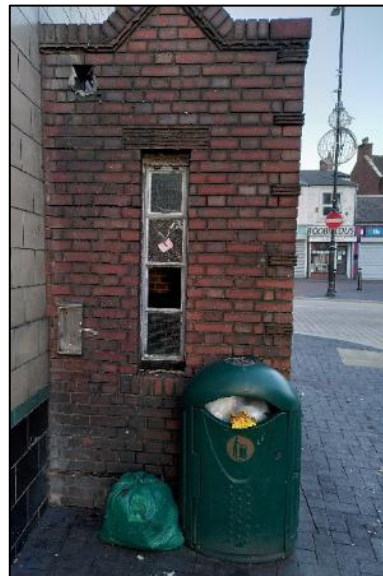
Figure 61 Former telephone Box, Side Elevation, Shambles.
