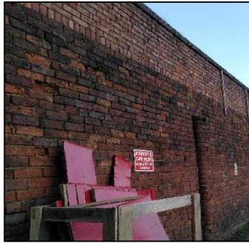
Figure 20 Wall, North of Shambles Car Park
