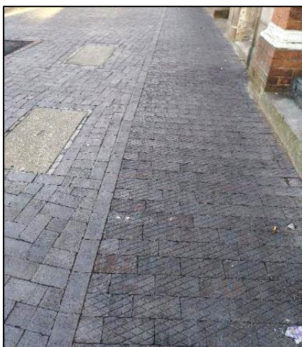
Figure 64 Blue diamond paving, Market Place
