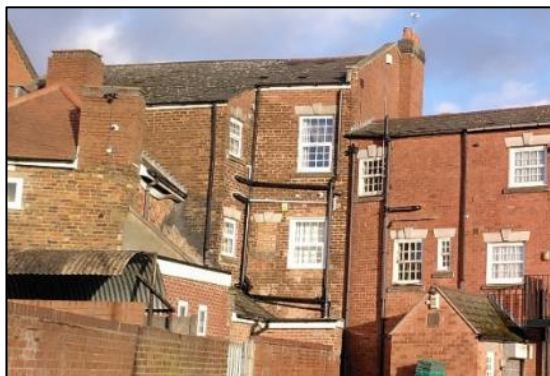
Figure 18 Rear of properties along Lower High Street
