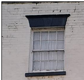
Figure 23 8/8 pane sash window, 32 Lower High Street
