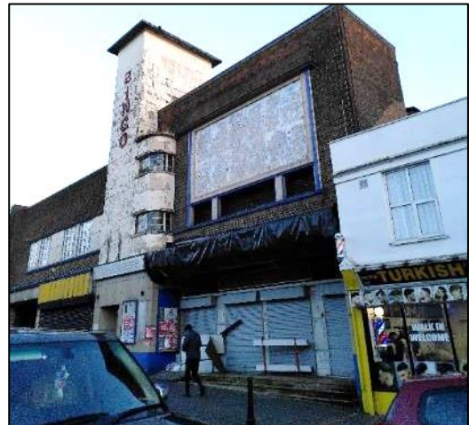
Figure 68 Locally listed former Gaumont Cinema, Walsall Street.
