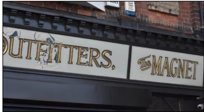
Figure 53 Former Outfitters, 13 Market Place
