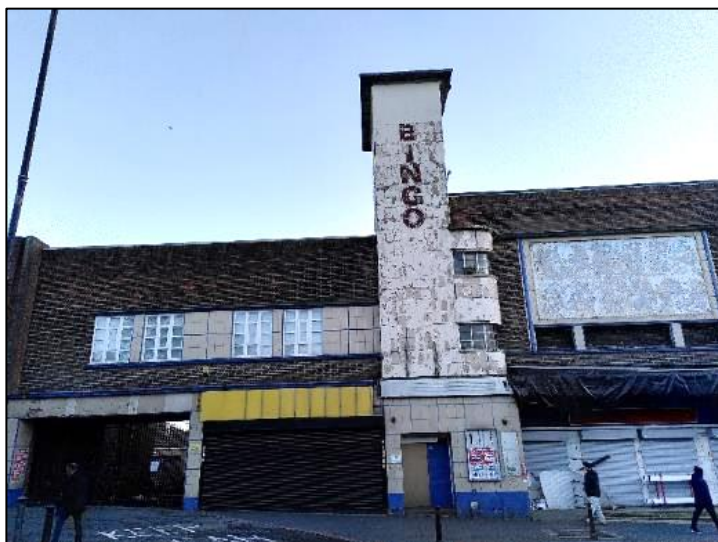
Figure 86 Former Cinema, Walsall Street
