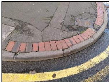
Figure 72 Paving Russell Street
