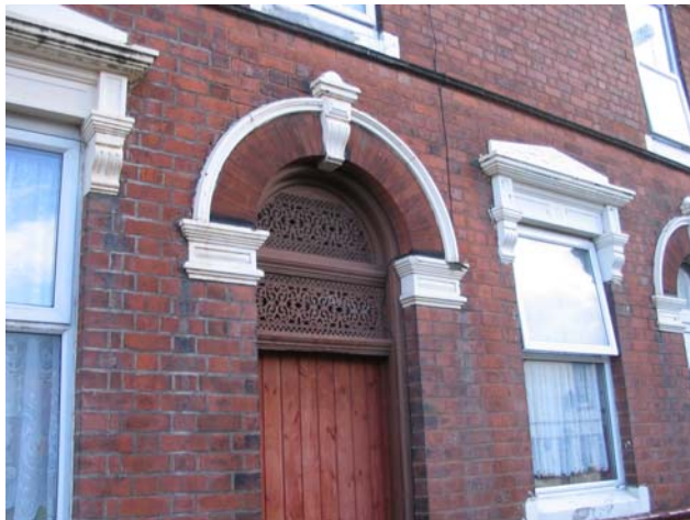
A typical cast ironwork fanlight.
