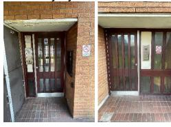
Each main (Front) entrance has a door entry system with a firefighter override switch.
