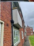
As part of a future works programme consideration should be given to replacing the staircase windows with windows that provide a larger opening window of 1m2 to aid smoke ventilation of the staircase.
