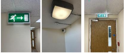
3) All installed lighting equipment is continually self-checked and connected by sim card to the installer. Any issues are highlighted to the installer who is contracted to make the necessary repairs.
