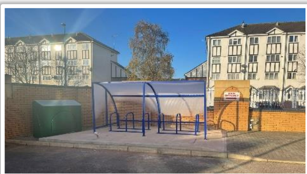
Figure 14- Bike stands installed at the Jamia Mosque, Smethwick
