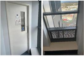
12)Communal windows can only be opened with the use of a key or by operating the automatic smoke vents.
