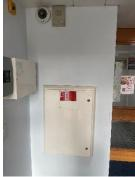
2) There is a dry riser that serves the building. The outlets are exposed and located on the communal lobby of each floor. Each exposed valve is secured with a cable tie. The caretakers check the cable tie is intact as part of their weekday inspections.
