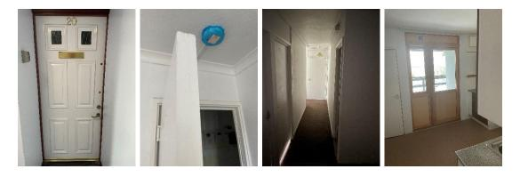
23) The panel above the fire door to the water heater cupboard does not appear to be fire resisting. The material should be confirmed and if required replaced with a 30-minute fire resisting board. This presents a low risk and can be incorporated within a future planned maintenance scheme.
