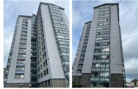
2) Each flat within the block has access to an individual winter garden balcony. These are cantilevered concrete floors with an aluminium and glass construction.
