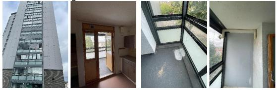
3) All windows are double glazed units housed in aluminium frames. Timber frames were noted internally within the staircase.
