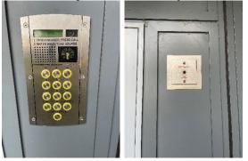
There is a firefighter's white box externally to the right -hand side of the main entrance to the front of the building. The box contains keys for the building and is secured with a bridge-door padlock.
