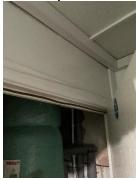
24) Flat 20 entrance door. The combined smoke strip to the frame on the slamming side of the door frame requires replacement.
