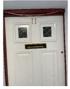
25) The lift doors at ground floor have no fire separation from the flats on the left-hand side of the building. The installation of a fire resisting door and partition should be considered as part of future works programme.
