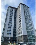
2) Each flat within the block has access to an individual winter garden balcony. These are cantilevered concrete floors with an aluminium and glass construction.
