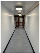
3) The means of escape from flats are dead ends. The un-ventilated corridors are less than 4.5 metres.
