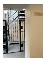
11) The chute room doors on each floor are 44mm nominal 30-minute fire doors with combined intumescent strips & cold smoke seals and overhead self-closing devices. The chute room on each floor has louvres to provide natural ventilation.
