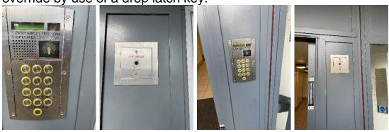
There is a firefighter's white box externally to the right -hand side of the main entrance to the front of the building. The box contains keys for the building and is secured with a bridge-door padlock.
