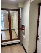
17) Service cupboards located within the corridors are 54mm nominal fire doors with intumescent strips and cold smoke seals secured with type 54 suited mortice locks.
