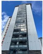
3) All windows are double glazed units housed in aluminium frames. Timber frames were noted internally within the staircase.
