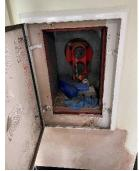
2) There is a dry riser that serves the building. The outlets are exposed and located on the communal lobby of each floor. Each exposed valve is secured with a cable tie. The caretakers check the cable tie is intact as part of their weekday inspections.
