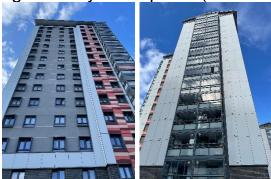
2) Each flat within the block has access to an individual winter garden balcony. These are cantilevered concrete floors with an aluminium and glass construction.
