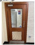
11) Glazing between the flatted accommodation and the staircase is in close proximity. Compensatory measures should be considered for a future works programme such as a sprinkler system to the flats.
