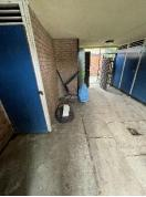
4) Natural smoke cross ventilation is provided by the "slated" construction on the front and rear facades of the bin store.
