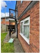
3) The front and rear façade and gates to the communal bin store area are timber. During the next planned future works programme consideration should be given to replacing the timber with a non-combustible
