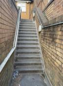
4. Both staircases lead to a 1<sup>st</sup> floor open deck access that's 1848mm wide.
