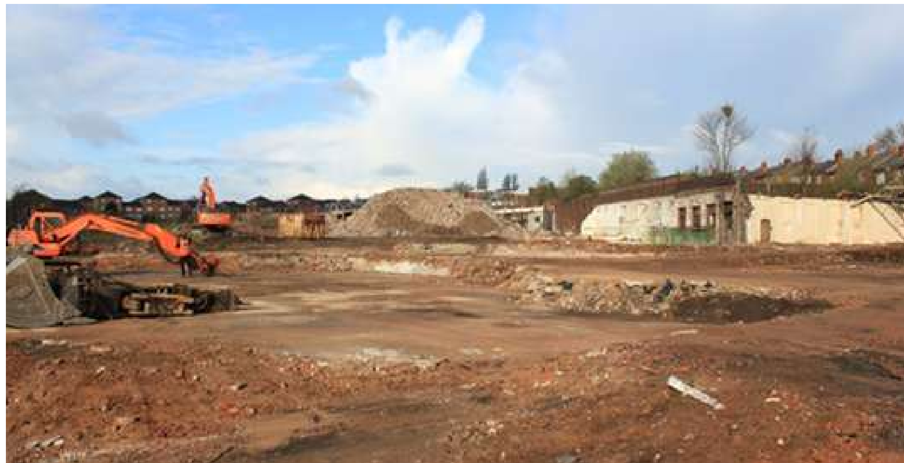
Site under construction (Source: Google)
