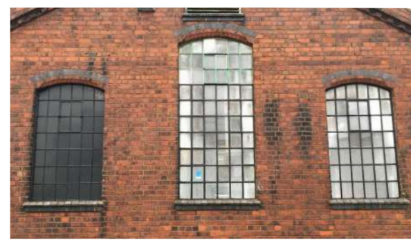
Buildings identified as architecturally significant along Bell Street.
