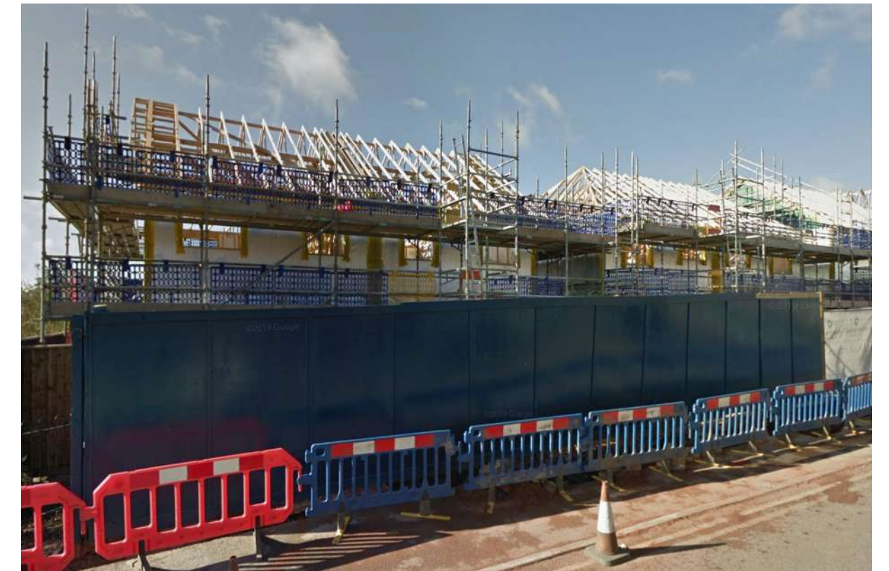
Site under construction (Source: Google)
