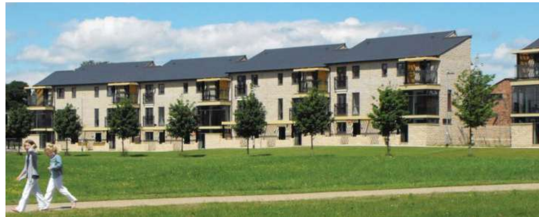
Two-storey houses facing public open space with car access and parking provisions at the rear, on Goldcrest Road (Source: Steve Tiesdell Legacy Collection)
