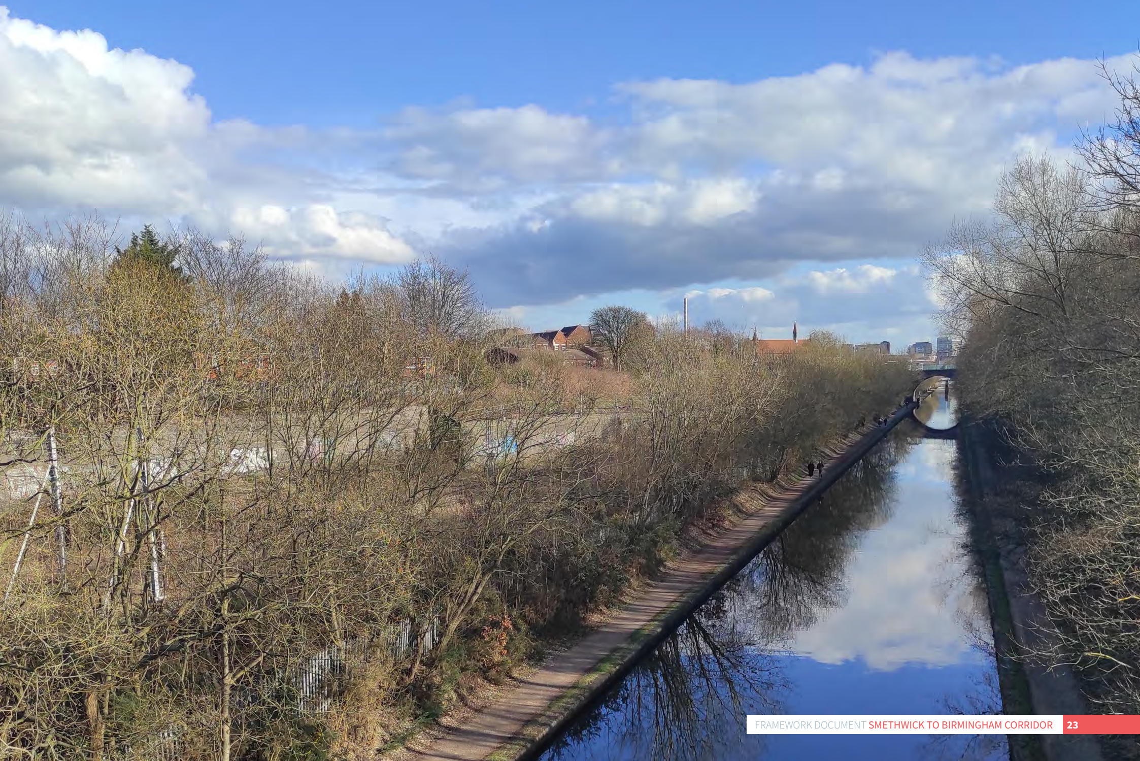
Fig. 3.11 - Typical view of the Main Line Canal through the corridor
