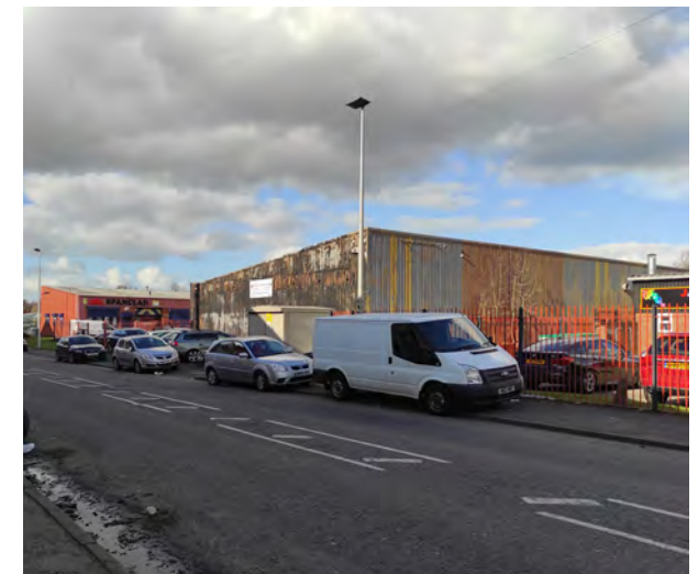
Fig. 3.10 - Typical industrial uses in the Grove Lane area
