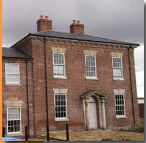
Listed building conversion Castle Street, Tipton
