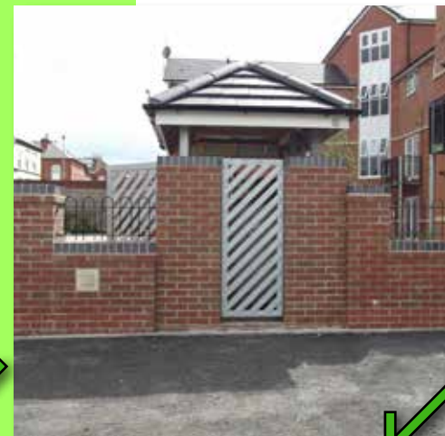
Bin storage must be well constructed and accessible.
