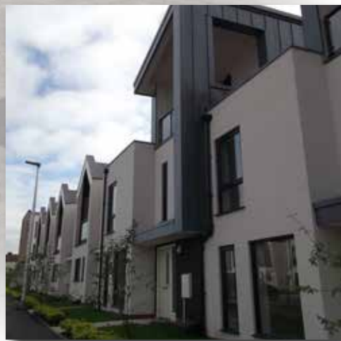
New homes, Eastern Gateway, West Bromwich. Accord Housing.
