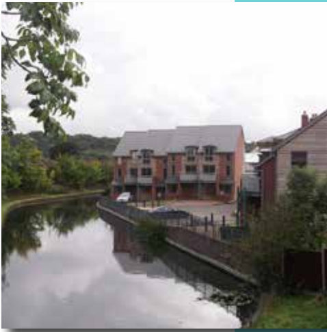
Canal Side Development, Castle Street, Tipton
