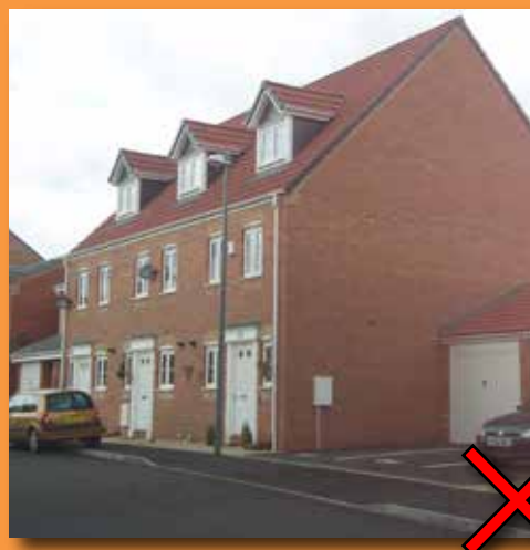
The lack of definition to front garden area, and exposed blank gable erodes the quality of the streetscene and impacts on the internal defensible space.
