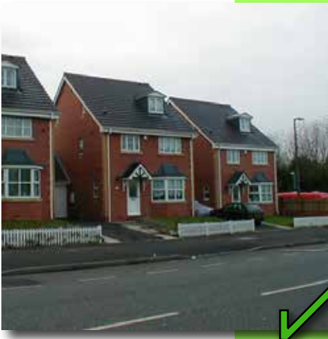
Car parking set back at the side of built form reduces the dominance of vehicles on the street frontage.
