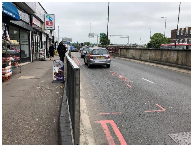
Photo 3 – Constrained footway and carriageway outside Perry Barr station, looking north
