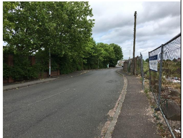
Photo 4 – Narrow footway, poor lighting and derelict unattractive route on Mill Lane
