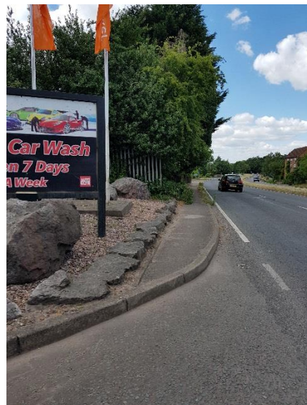
Photo 6 – Narrow footway without dropped kerbs on access to garage on A452
