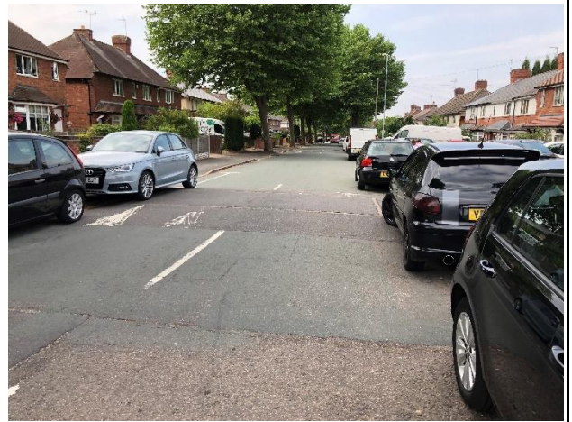
Photo 4 – Existing traffic calming and 20mph speed limit on Leighswood Avenue, but constrained opportunity to provide cycle infrastructure due to on street parking
