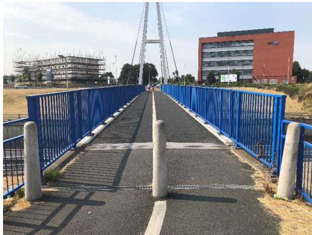
Photo 9 – Segregated footway/cycle on bridge over The Expressway A41
