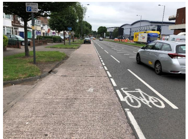
Photo 4 – Existing advisory cycle lane on the outside of parking bays on the A34 north of Cliveden Avenue
