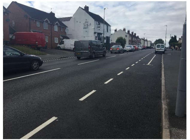
Photo 14 – On-street parking bays on A4196
