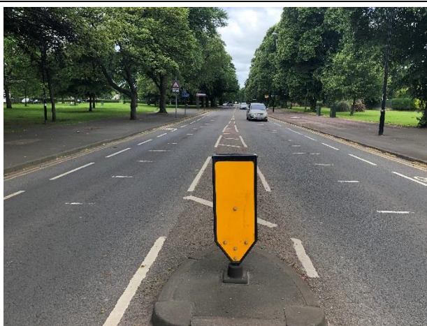
Photo 5 – Wide carriageway and existing mandatory cycle lanes on both sides of Binley Road
