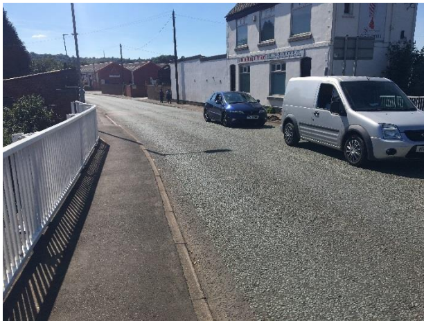
Photo 1 – Biddings Lane, bridge over canal
