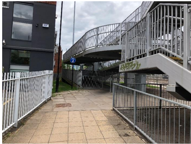
Photo 3 – Existing pedestrian and cycle bridge crossing the ring road between Hill Street and Upper Hill Street
