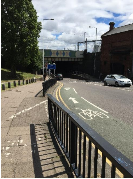
Photo 1 – Existing constrained and unclear cycle provision on the A4124 close to the ring road approaching the railway bridge
