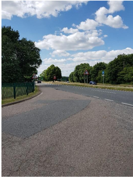
Photo 7 – No existing pedestrian or cycle provision on access and egress to garden centre. High vehicle speeds, but wide central reservation to re-align carriageway and accommodate pedestrian/cycle provision
