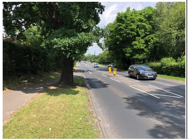
Photo 10 – Mature trees on the verge of Clifford Bridge Road may constrain alignment of cycle provision
