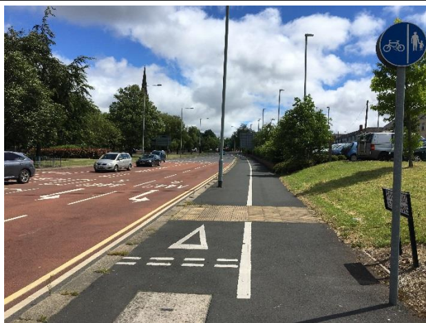
Photo 5 – Existing segregated cycle lane on south side of the ring road
