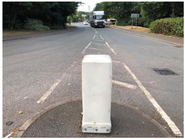
Photo 2 – Wide carriageway width near the junction of Wharf Approach and Stubbers Green Road, but level of HGV traffic is intimidating for cyclists. Segregation recommended
