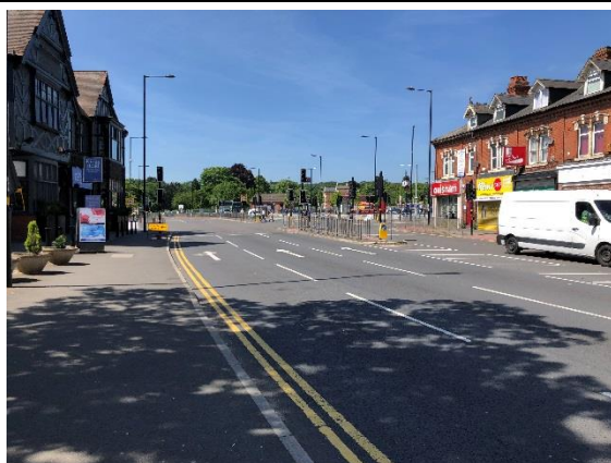
Photo 1 – A456 Hagley Road / A4040 Lordswood Road Junction (Bearwood) looking westbound
