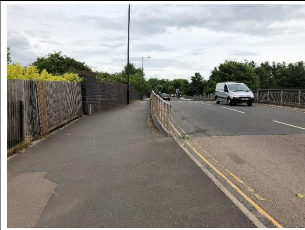
Photo 9 – Constrained width across railway and road bridge on Lythalls Lane
