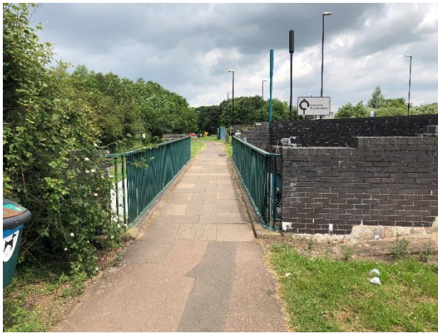
Photo 9 – Constrained footbridge on Clifford Bridge Road, crossing the River Sowe
