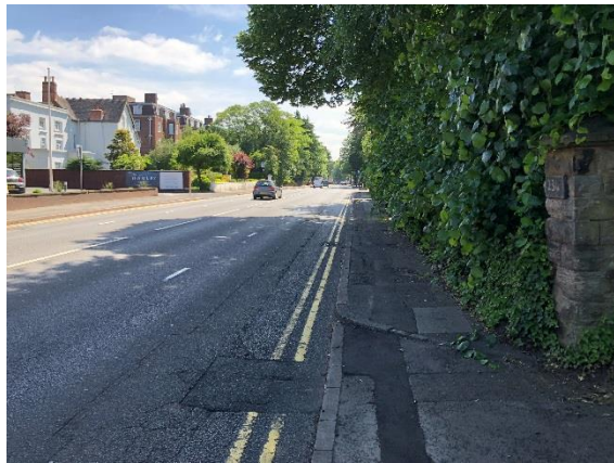
Photo 3 – Narrow footway on south side of A456 carriageway between Hermitage Road and Westfield Road looking eastbound
