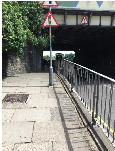
Photo 2 – The constrained footway and carriageway under the railway bridge on A4124
