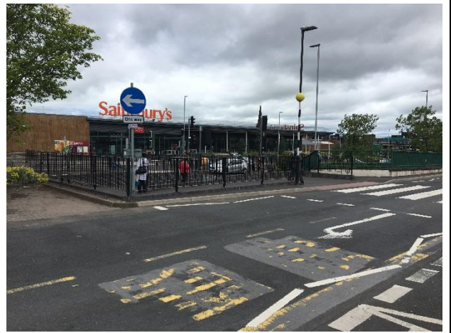
Photo 2 - Existing crossing on Peel Street, parking area and ring road, requiring cyclist to dismount
