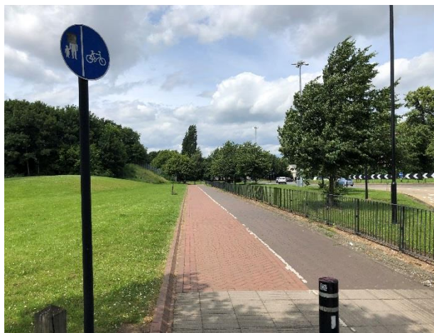
Photo 3 – Existing off-carriageway segregated footway/cycleway to the south of the Sky Blue Way/A444/Binley Road roundabout junction
