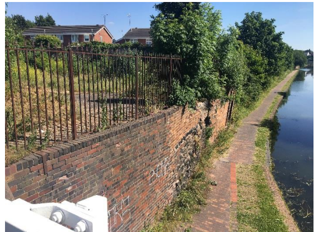
Photo 2 - Canal towpath looking south from Biddings Lane Bridge
