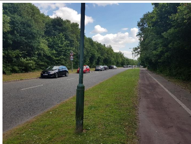
Photo 2 – Existing light segregated footway/cycleway on Hallmeadow Road. Wide carriageway and verge, but with on-street parking
