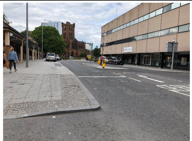
Photo 2 - Existing wide carriageway and footway but with parking bays on Queen Victoria Road
