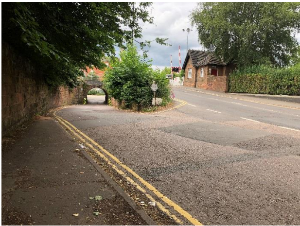
Photo 5 – Railway level crossing and alternative underbridge at Coundon Road and Barker's Butts Lane
