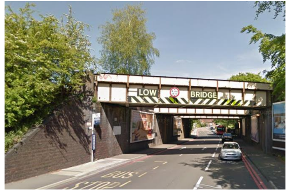
Photo 8 – Constrained footways and 3 traffic lanes under the railway overbridge close to Solihull town centre
