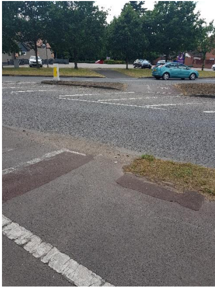
Photo 3 – Existing faded informal footway/cycleway crossing at the A452 / Hallmeadow Road junction
