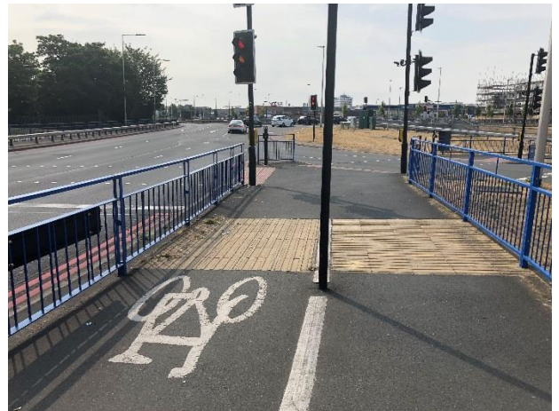
Photo 10 – Existing toucan crossings and segregated footway/cycleway at the All Saints Way / A41 junction
