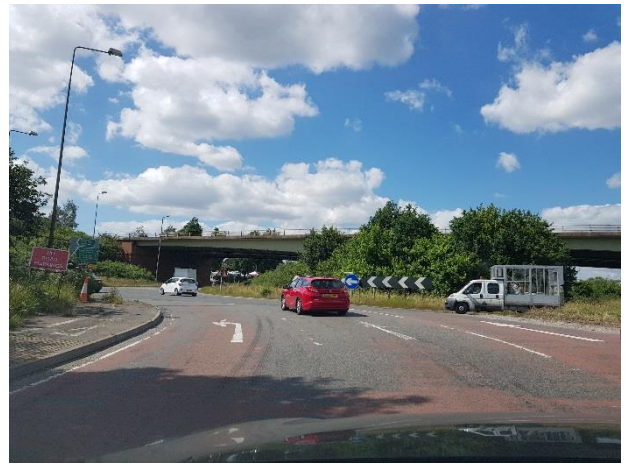
Photo 12 – Existing isolated footway/cycleway provision on west side of A452/A45 junction
