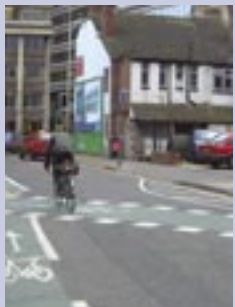
Cambridge One-way cycle contra-flow should not end prior to hazardous bend.
