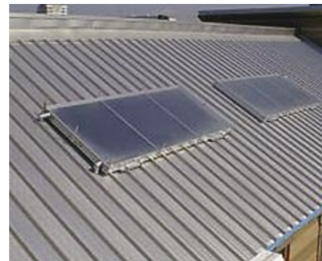
FIGURE 27 - SOLAR WATER HEATING PANELS - INTEGER HOUSING PROJECT
