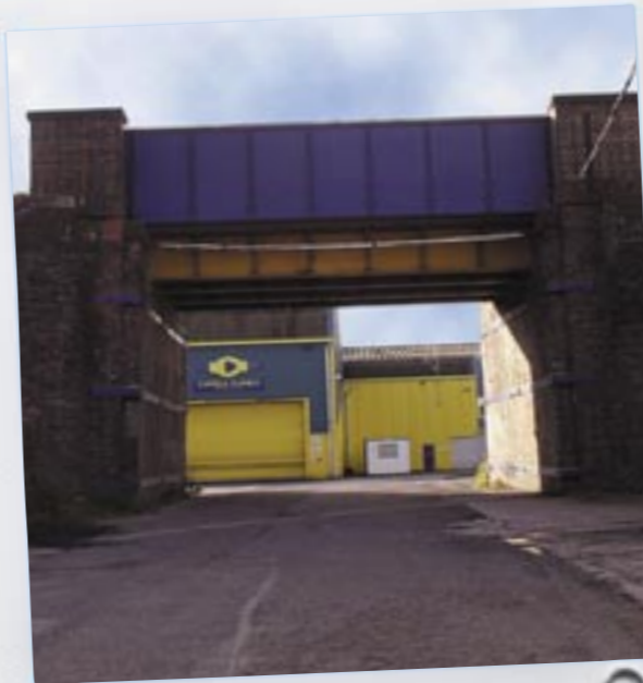
Poor pedestrian access and lack of natural surveillance in older developments.
