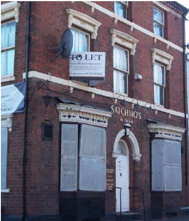
Vacant Public House, Old Hill
